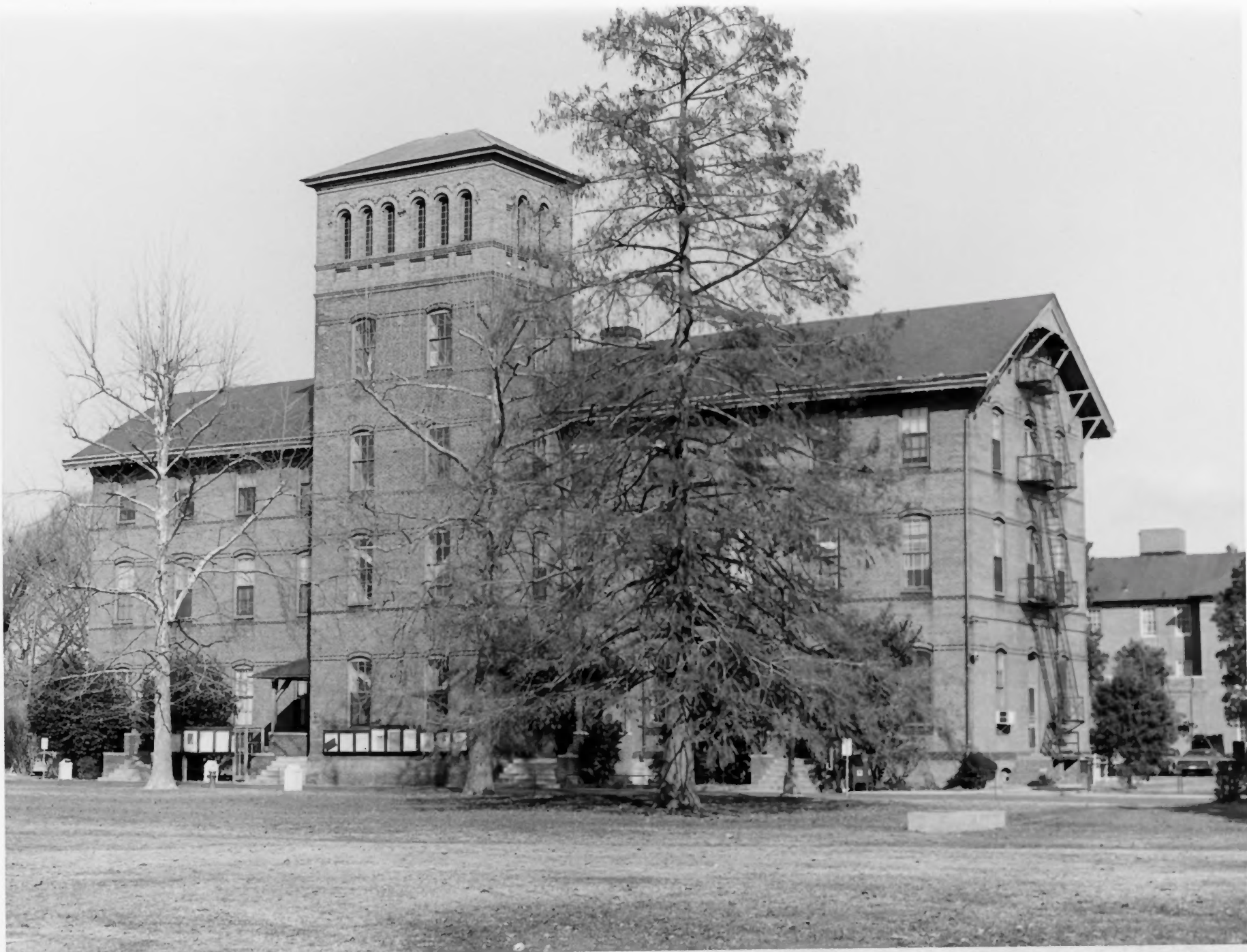
Stone Building, Hampton Institute, Hampton, Virginia
