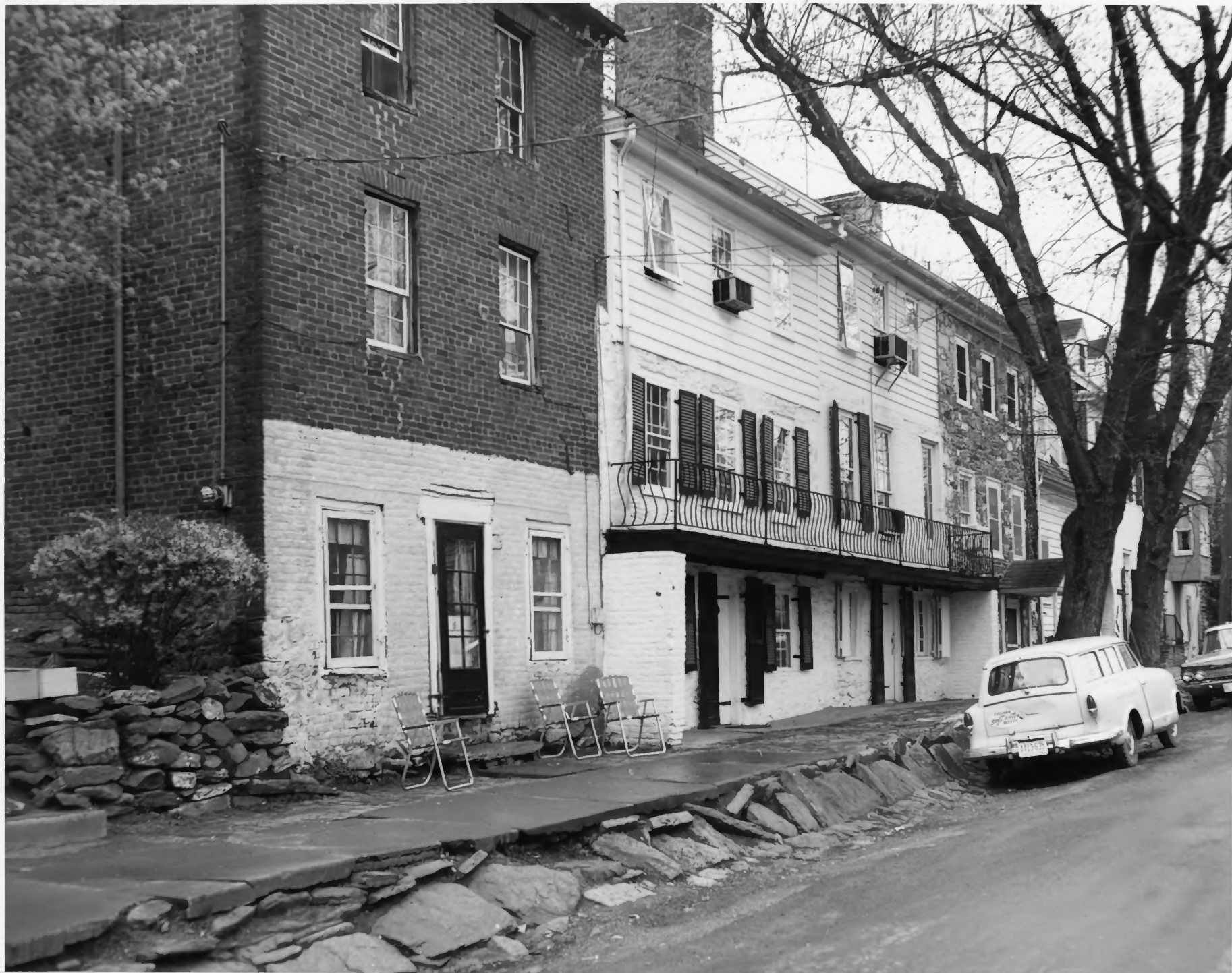
North side of Main Street, Waterford, Virginia
