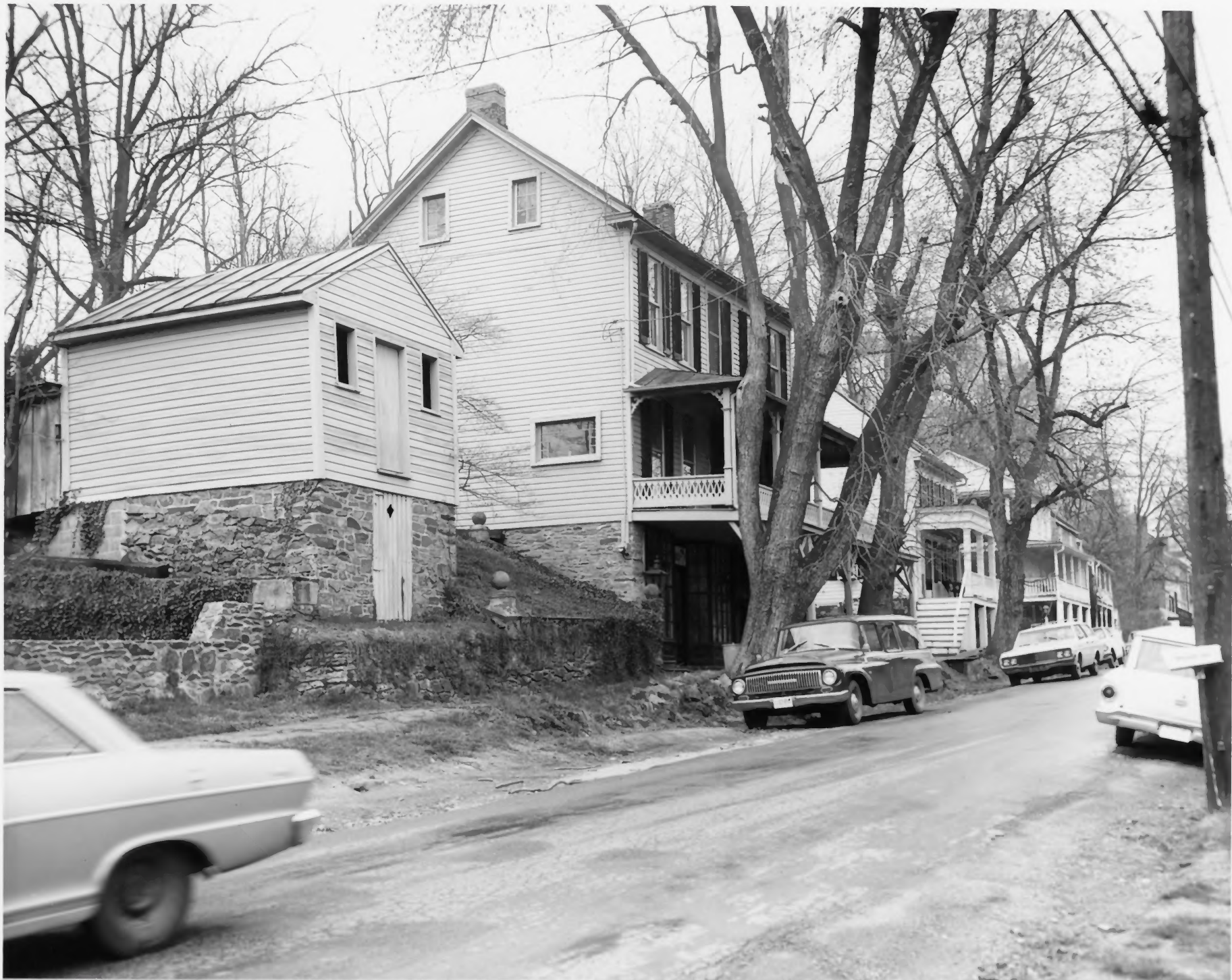
North side of Main Street, Waterford, Virginia
