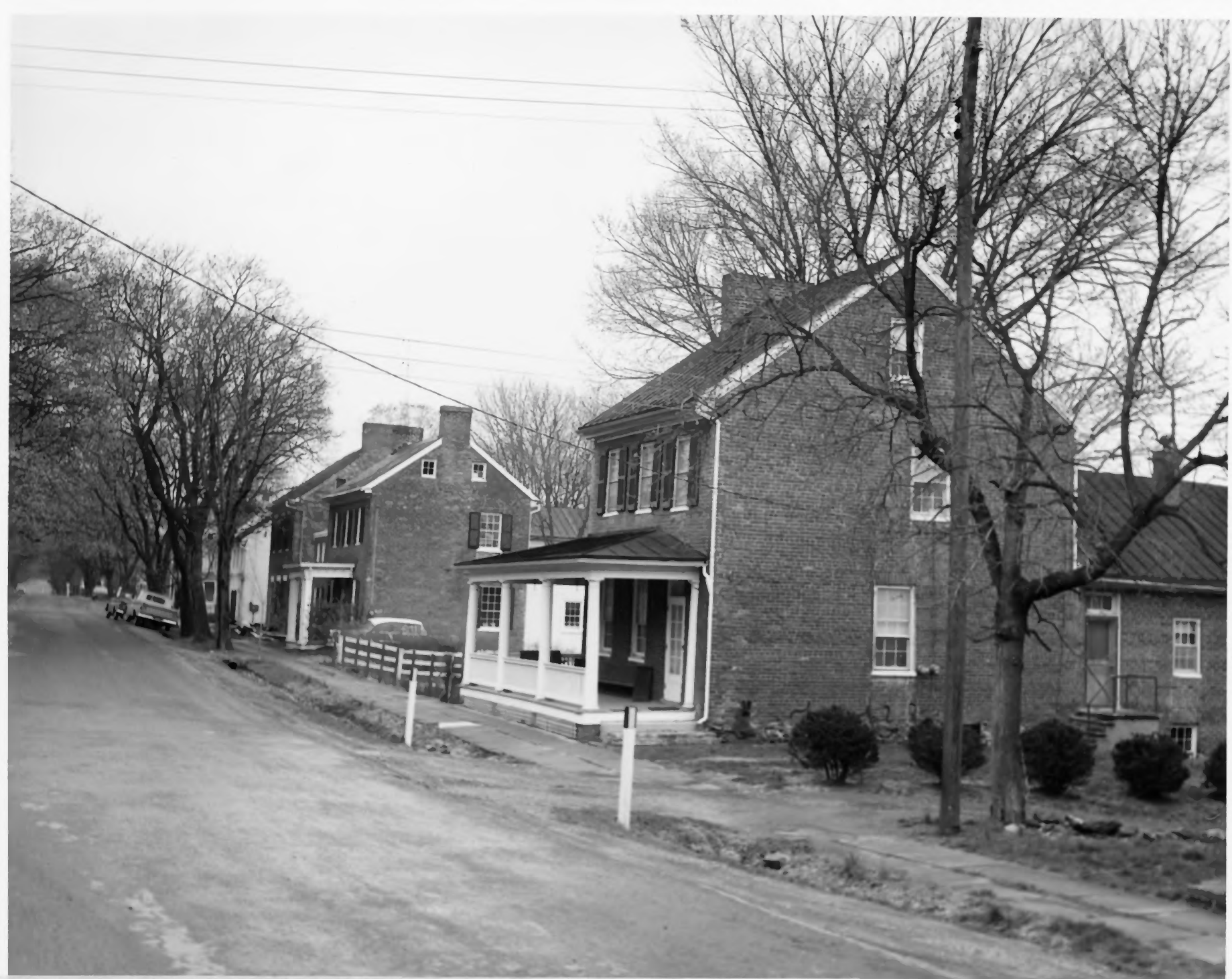
West side of Second Street, Waterford, Virginia
