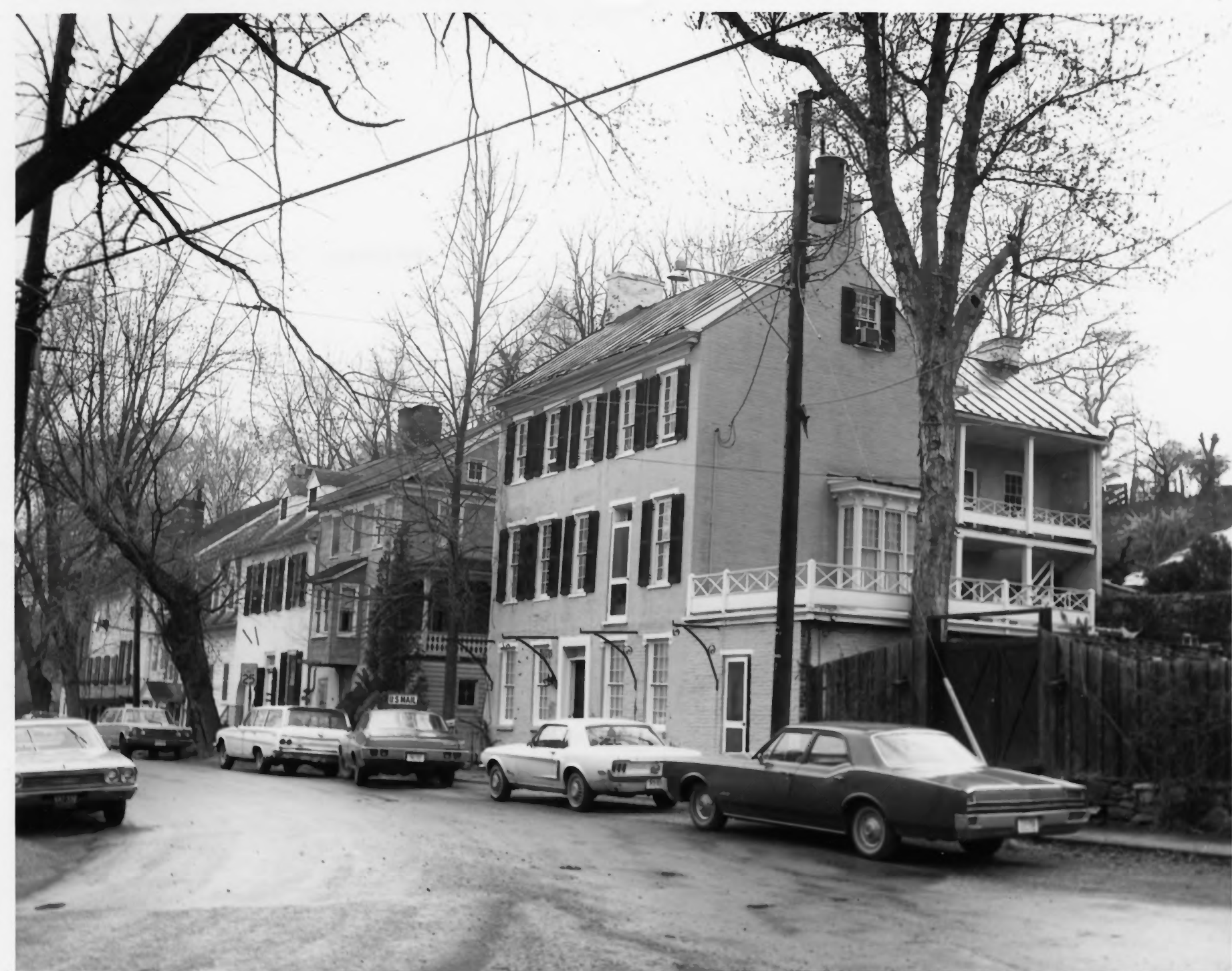
North side of Main Street, Waterford, Virginia
