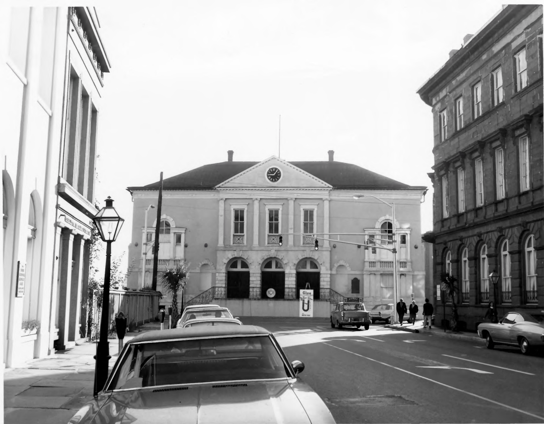
The Exchange and Provost--West and present front elevation, Charleston, South Carolina
