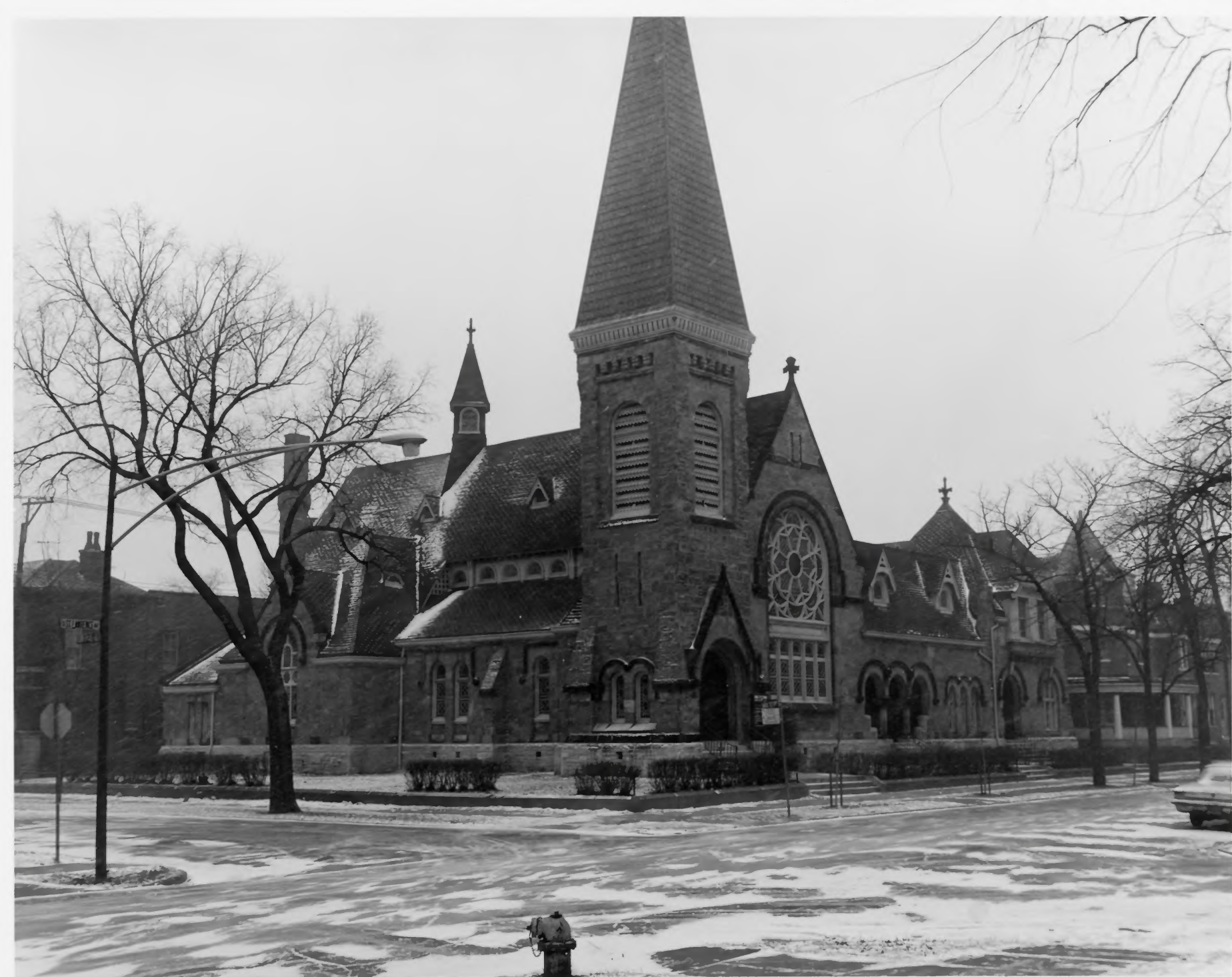
Greenstone Church - Pullman Historic District, Chicago, Illinois
