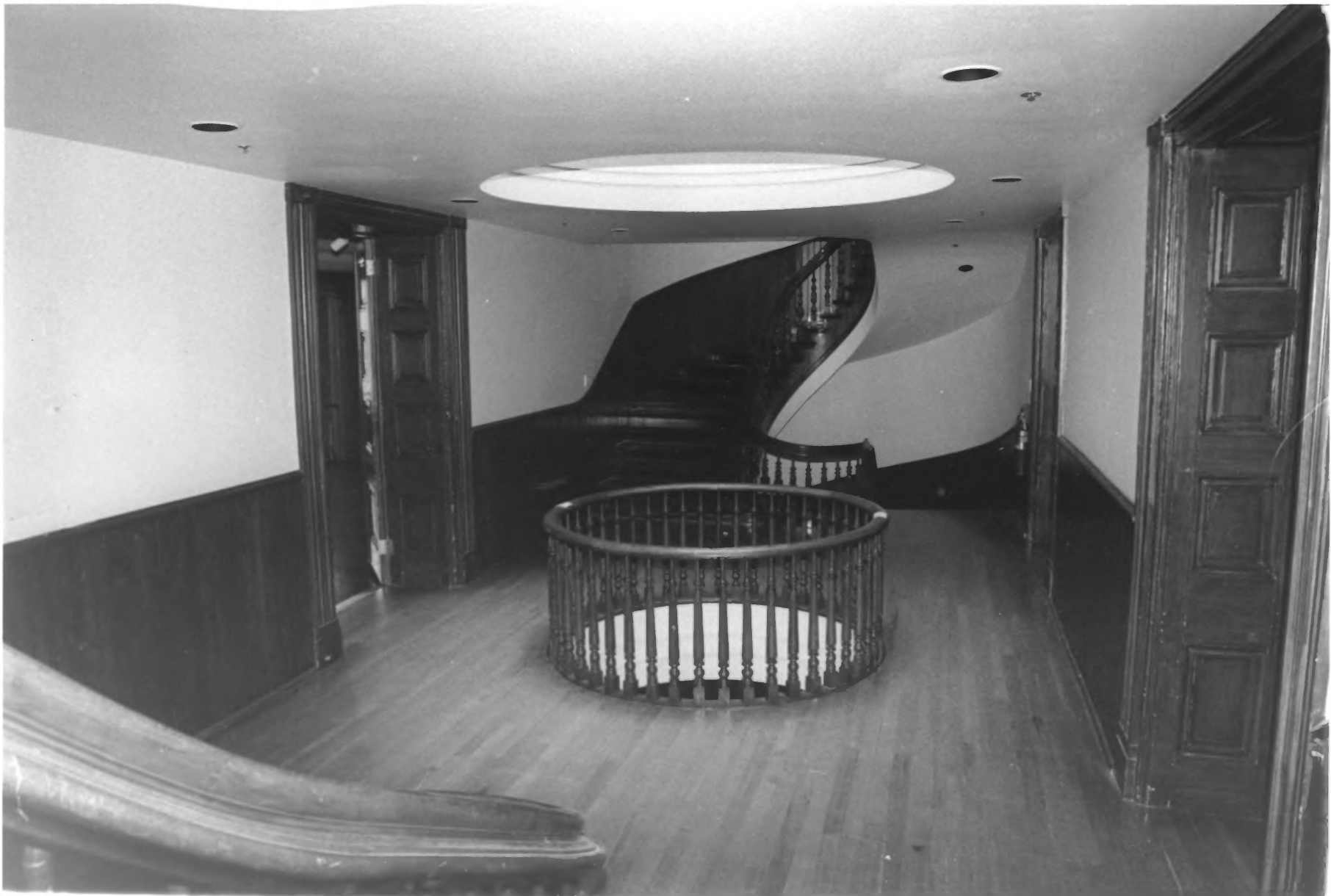
OLD STATE HOUSE Little Rock, Arkansas Central temple, 2nd floor hall Photo by R. Logan, 9/96
