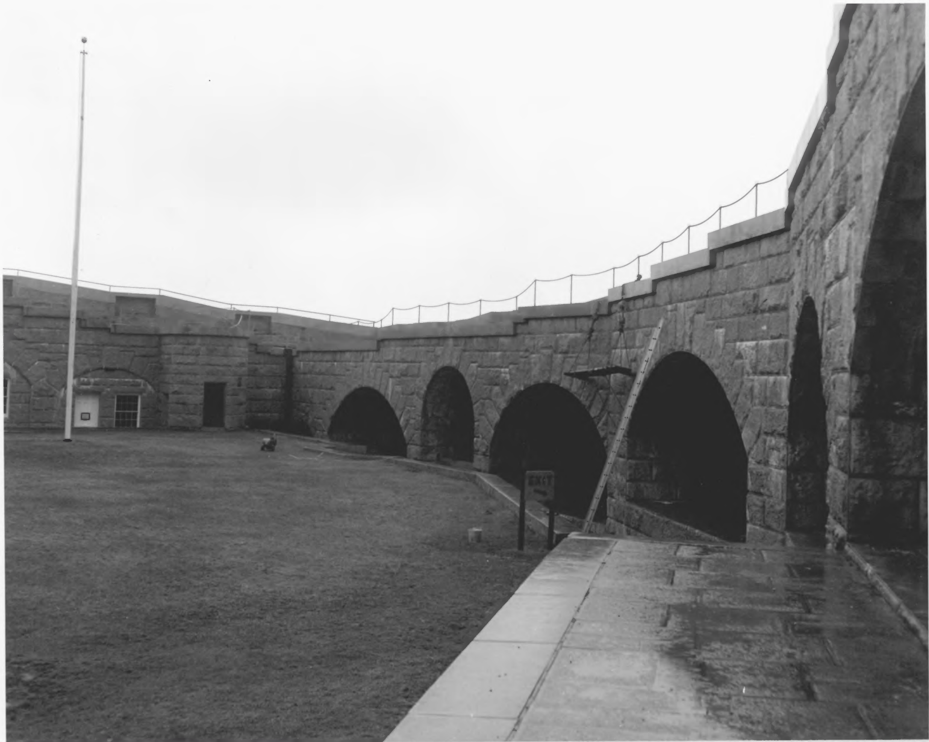
Fort Knox, Maine. Casemates in river wall and parade ground.
