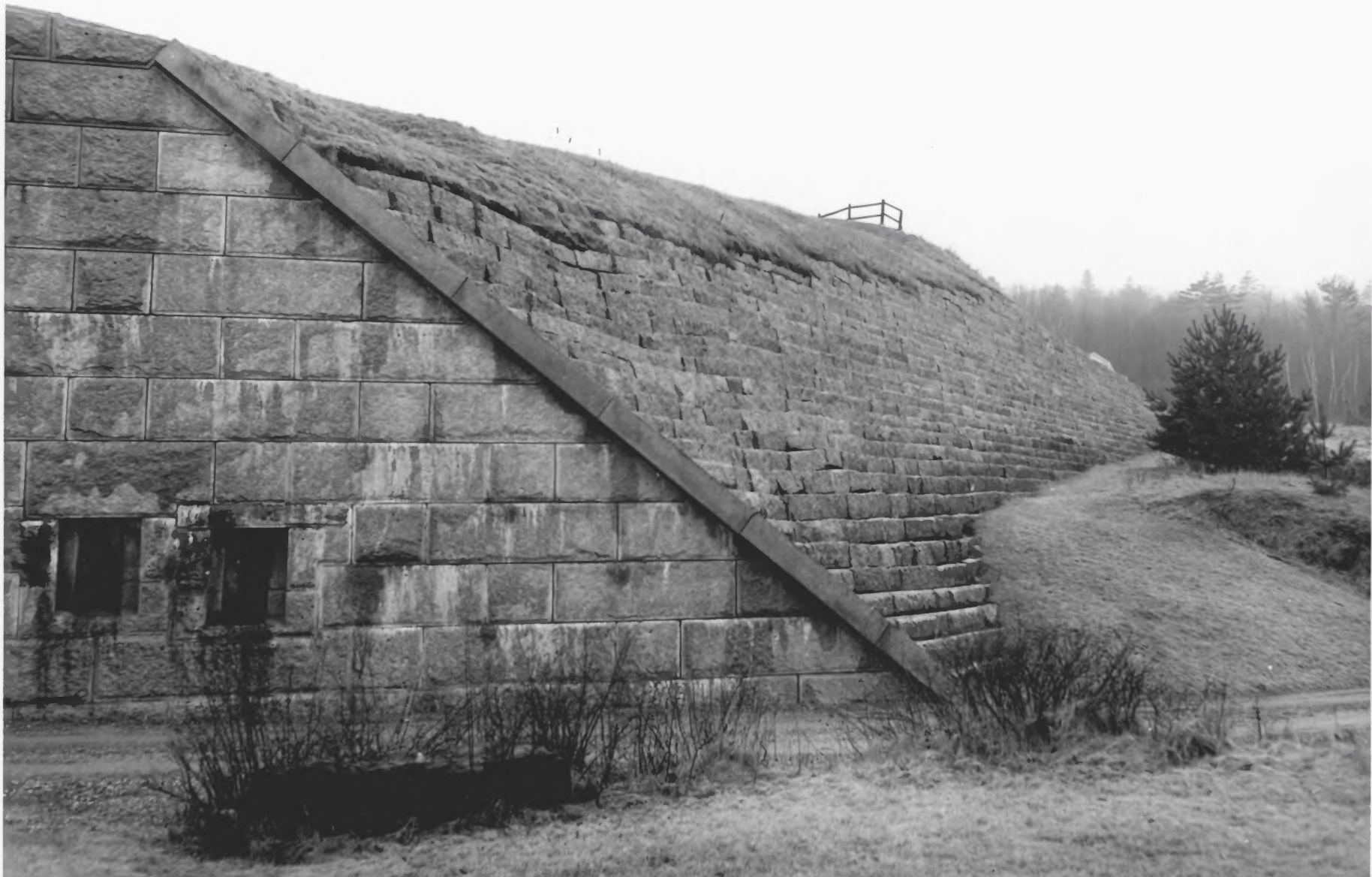
Fort Knox, Maine. Granite eastern end and outer facing of north earthen wall. NPS Photo 1970
