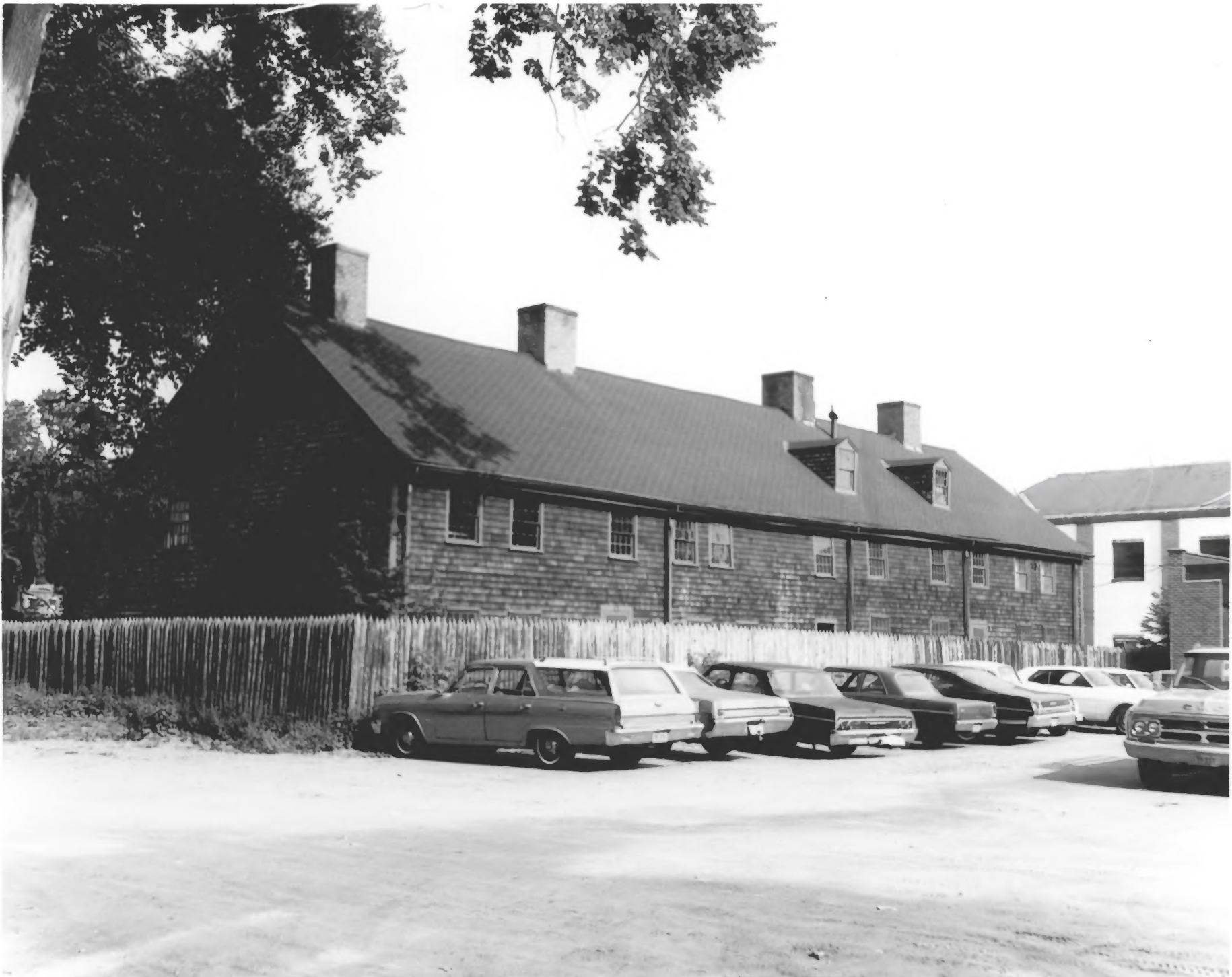
Fort Western, Augusta, Maine Rear elevation.
