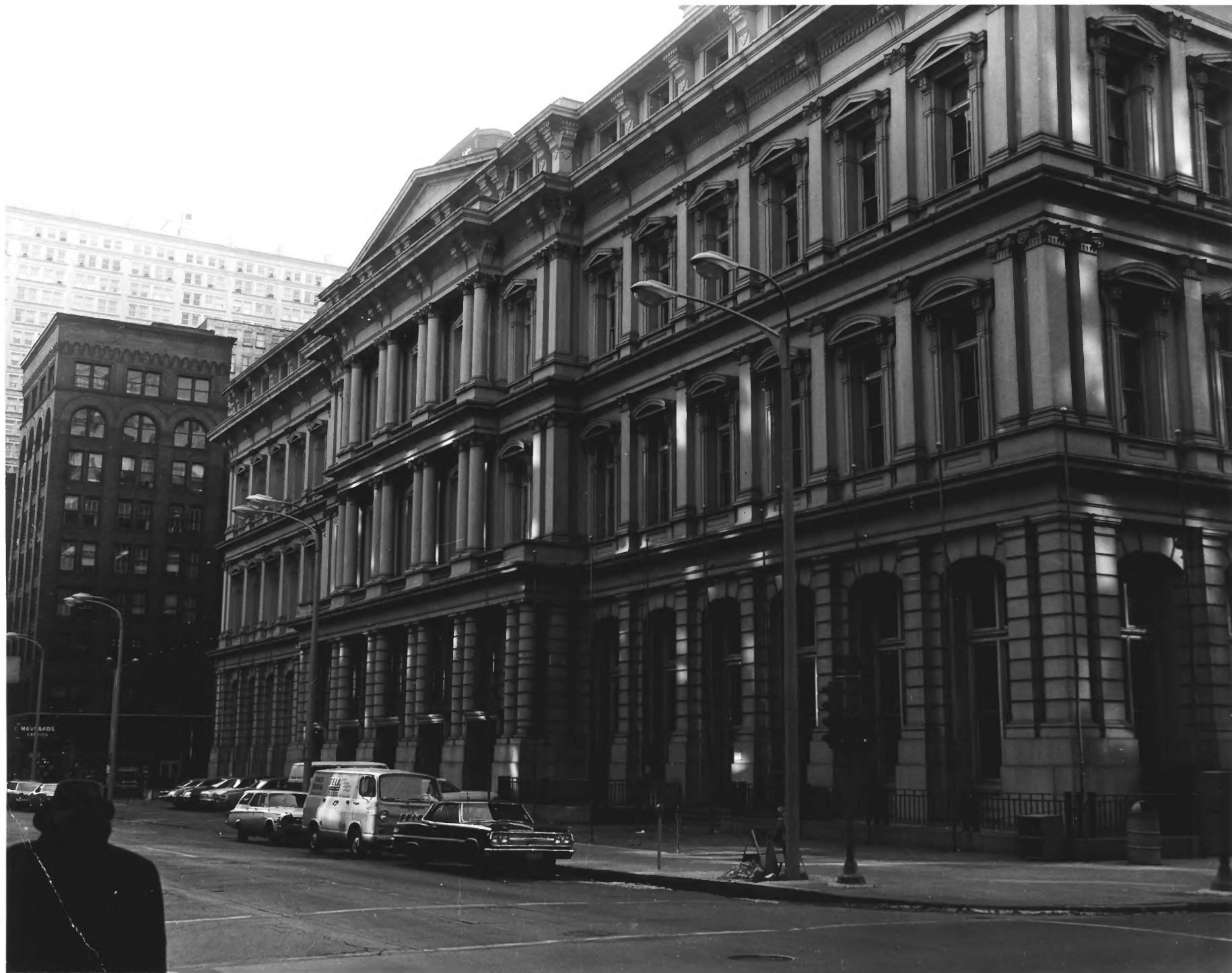
13 Old Post Office (Rear elevation), St. Louis, Missouri
