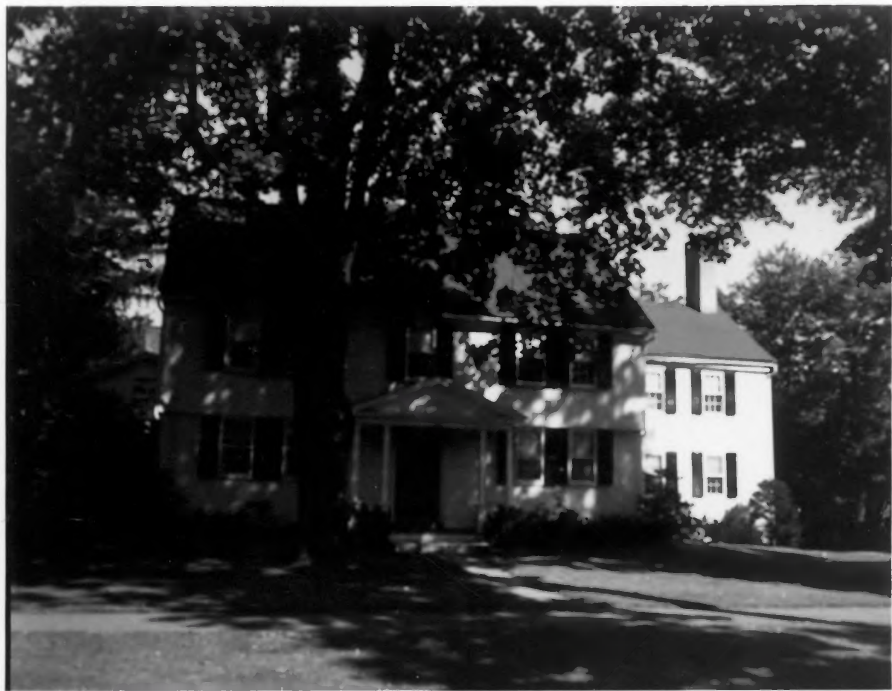
Oliver Wolcott, Sr. House, 1753 South Street
