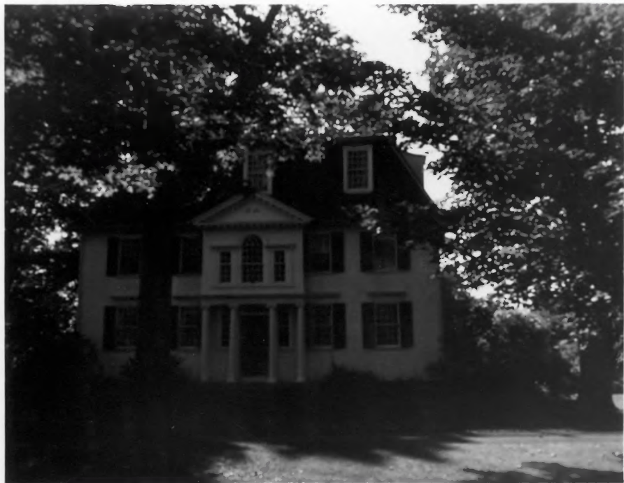
Sheldon's Tavern, 1760 North Street Iitchfield, Connecticut
