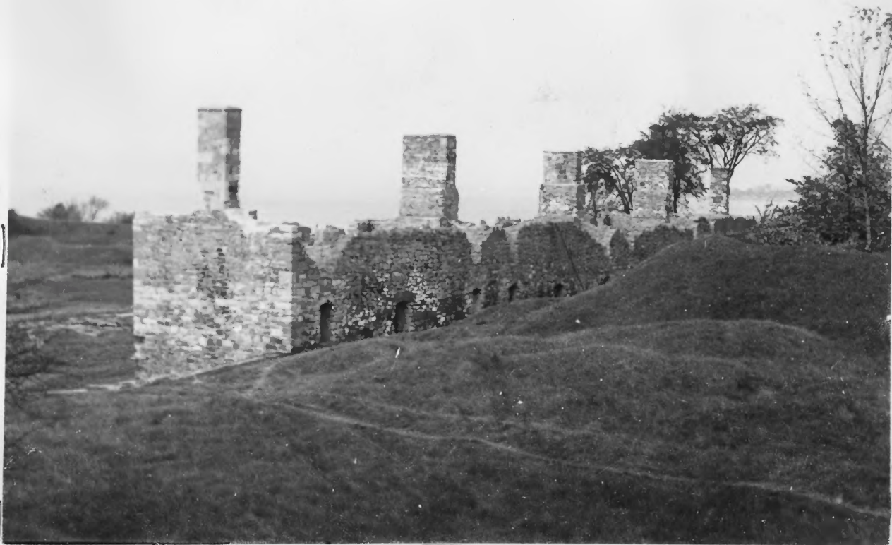
VIEW OF BARRACKS SHOWING CHIMNEYS STILL STANDING
