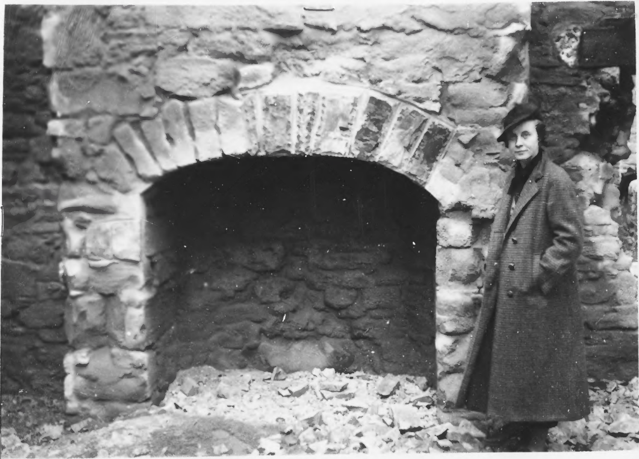
CLOSE-UP OF FIRST FLOOR FIREPLACE
