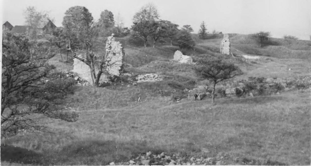
OLD CHIMNEY STACKS, ALL THAT IS LEFT OF THIS SECTION OF BARRACKS
