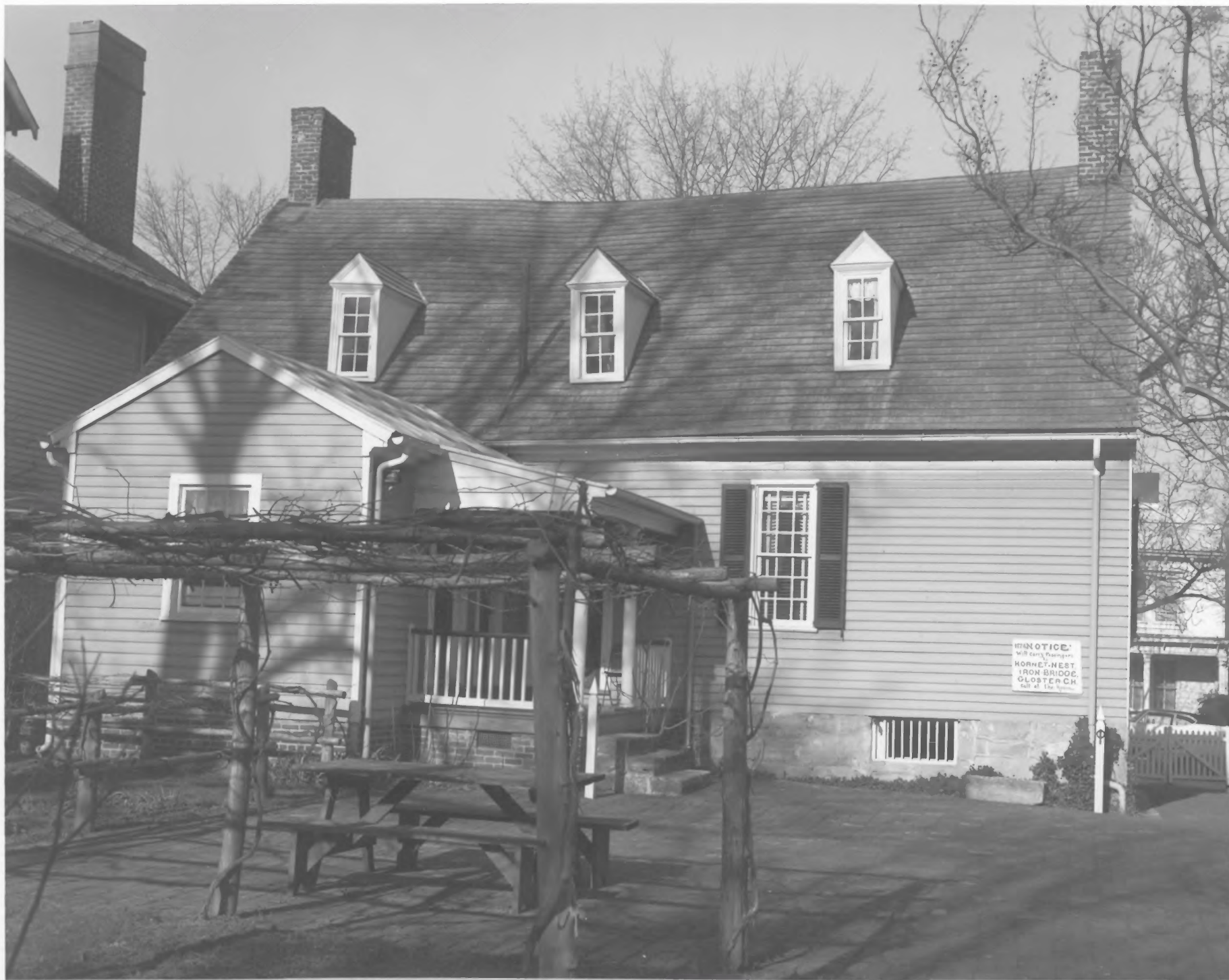
Rising Sun Tavern, Fredericksburg, Virginia, Rear (West).
