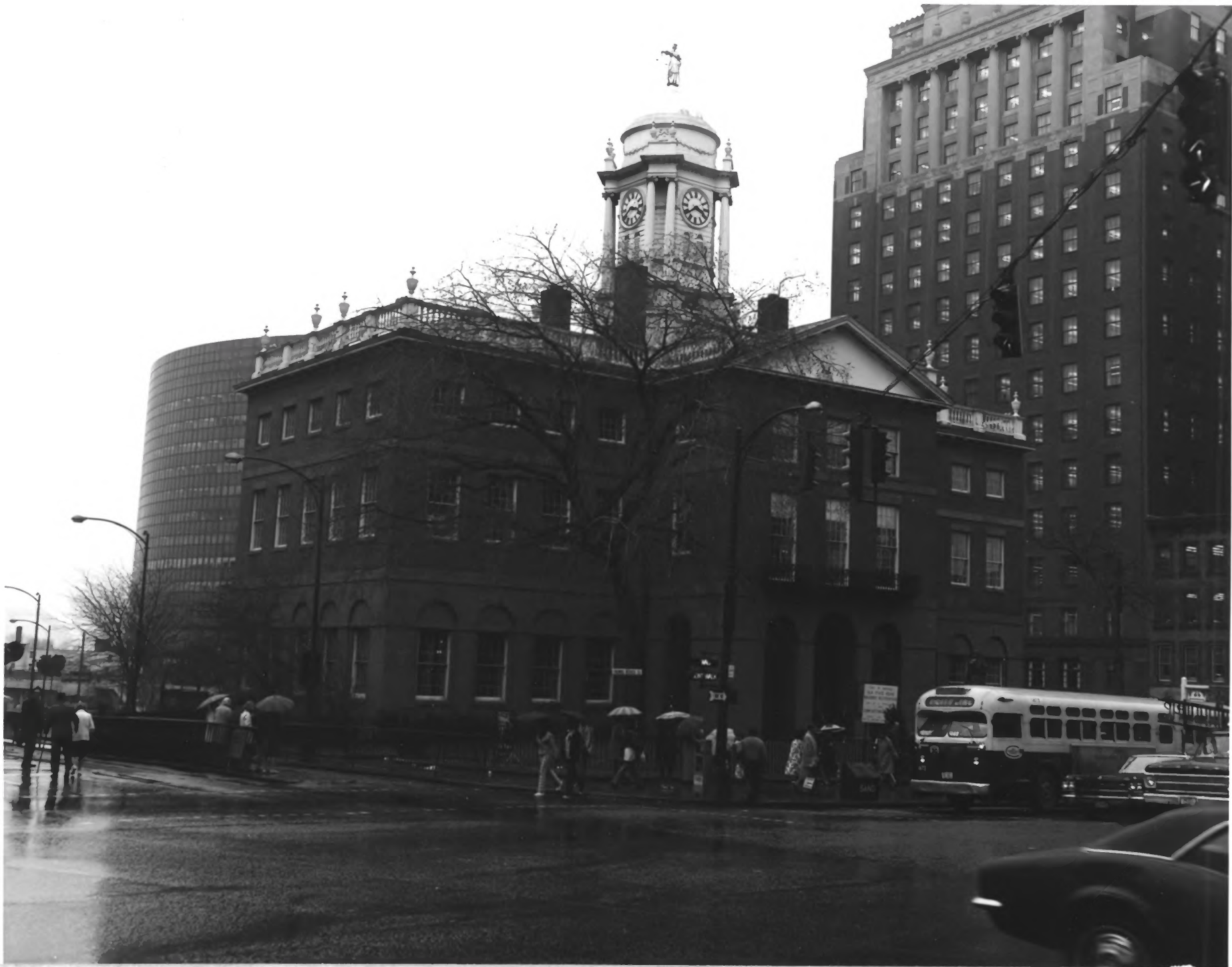
Old State House, Hartford, Connecticut (West elevation)
