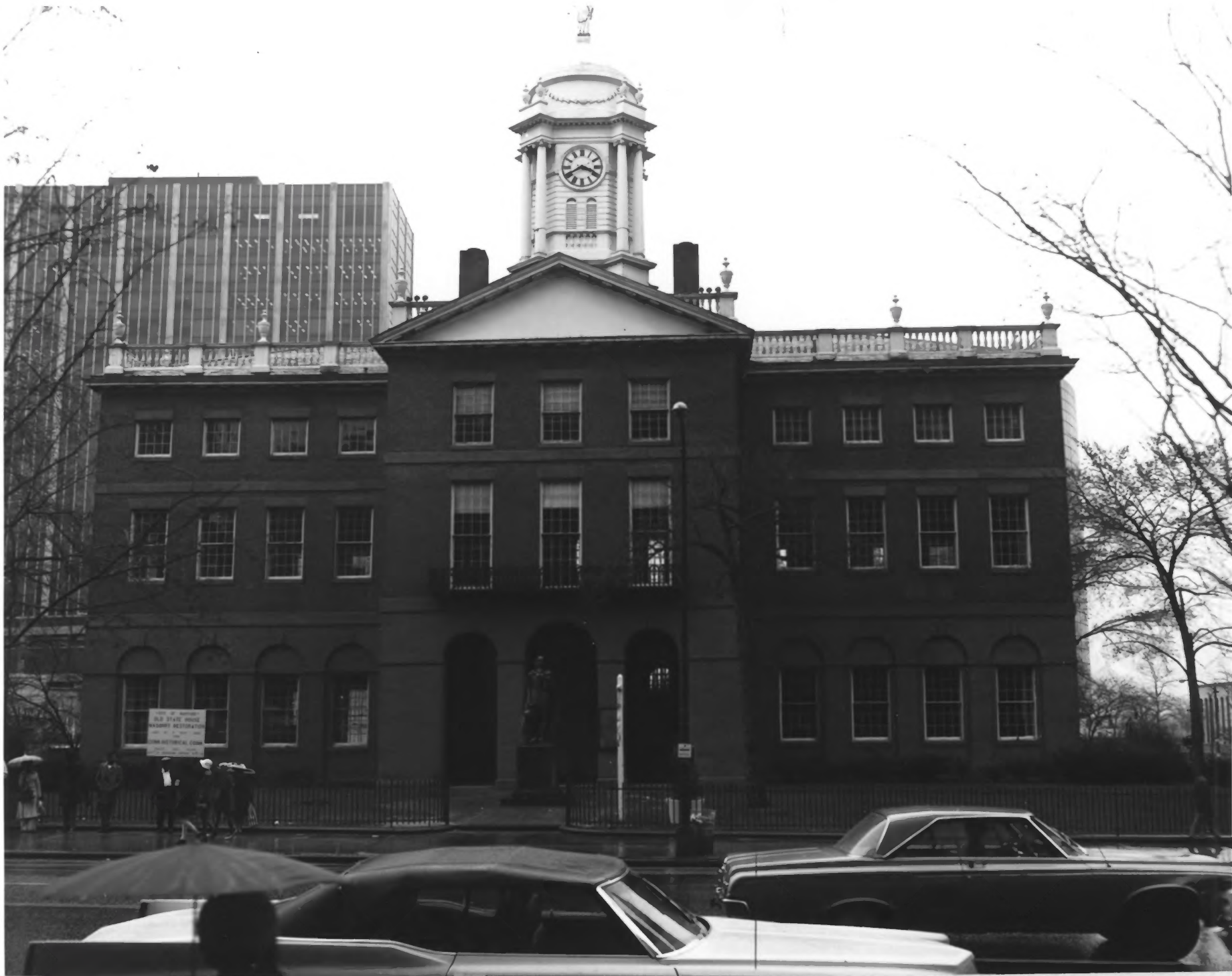
Old State House, Hartford, Connecticut (west elevation)
