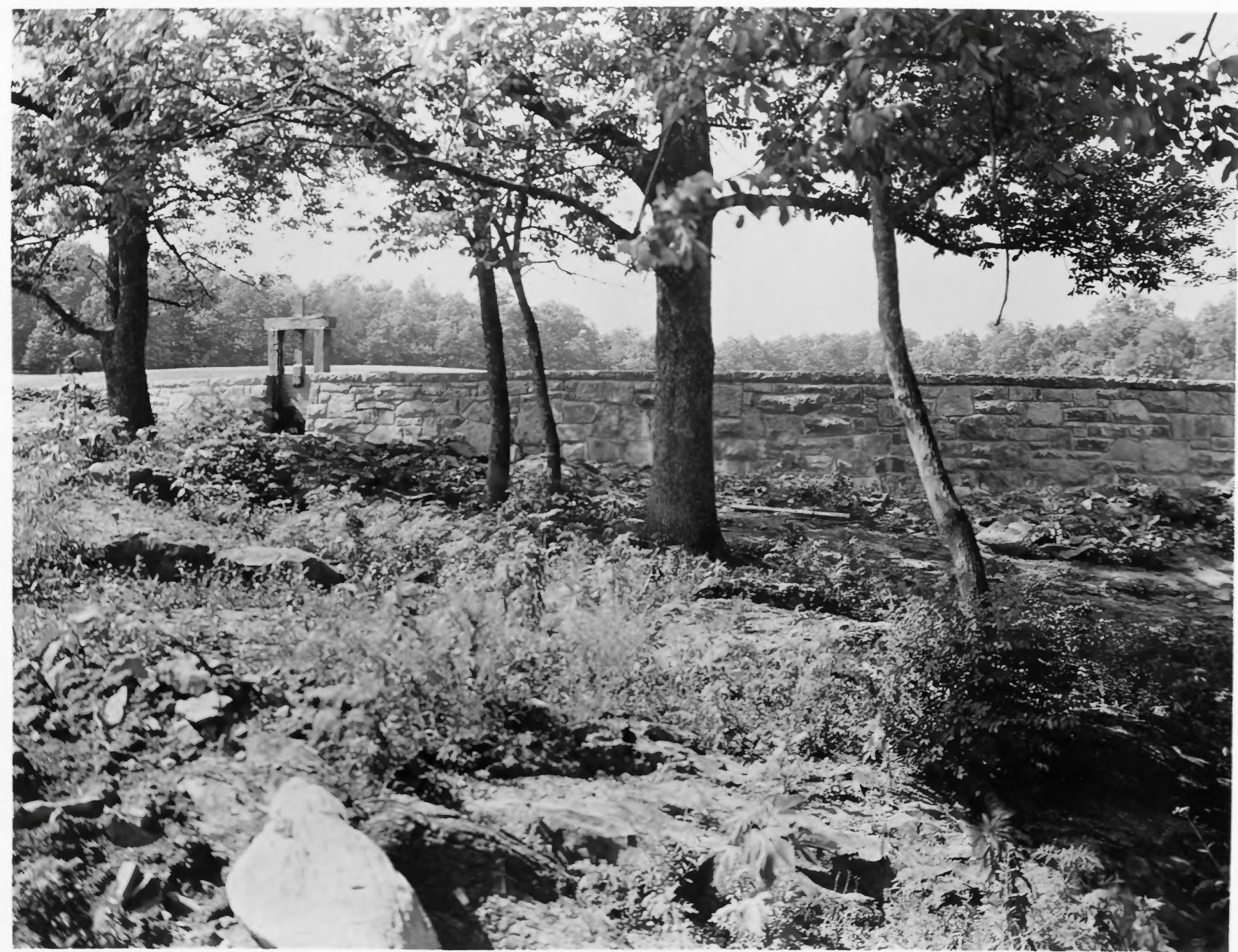
View of left end of Dam Wall, showing Headgate for Race.
