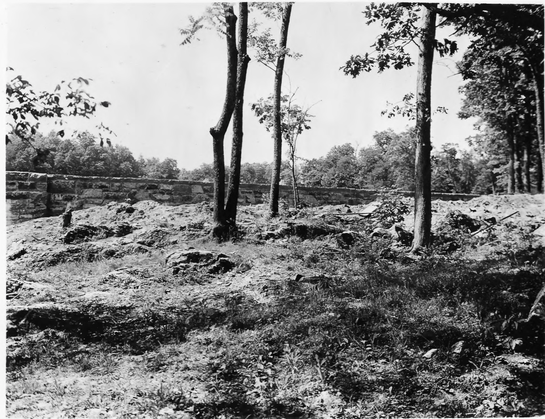
View of outside of Dam at right end.
