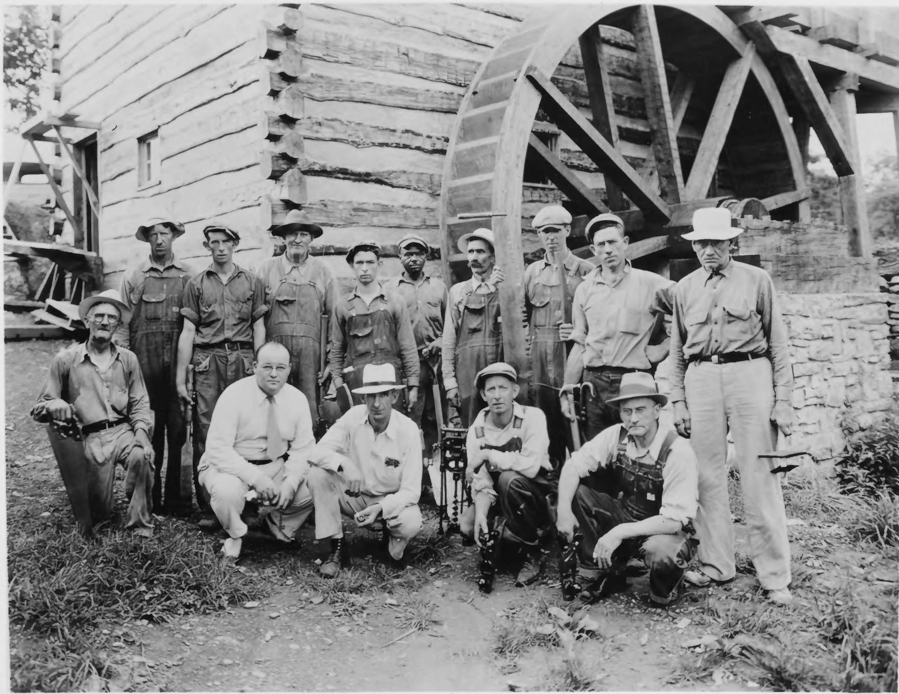
H. A. Kellar with Foreman, A. L. Oviatt, and a picked group of workmen, skilled in working with wood, stone, and iron, who did the most difficult parts of the restoration of the Race, Mill, Mill Machinery and Slave Cabin.
