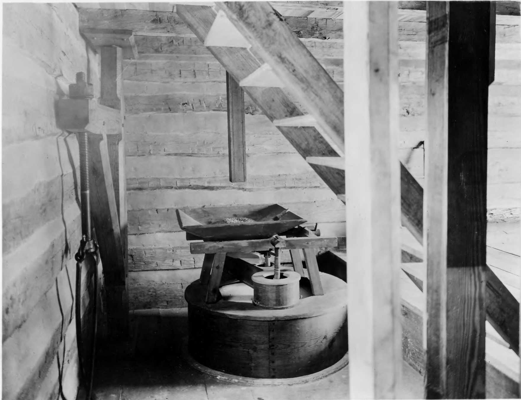
5. Corner of Mill, Second Floor, showing Corn Burrs and Apparatus. Note on left the Crane used to raise and lower the stones for sharpening. On the right, stairway to Third Floor. Right foreground note Elevator Chutes.
