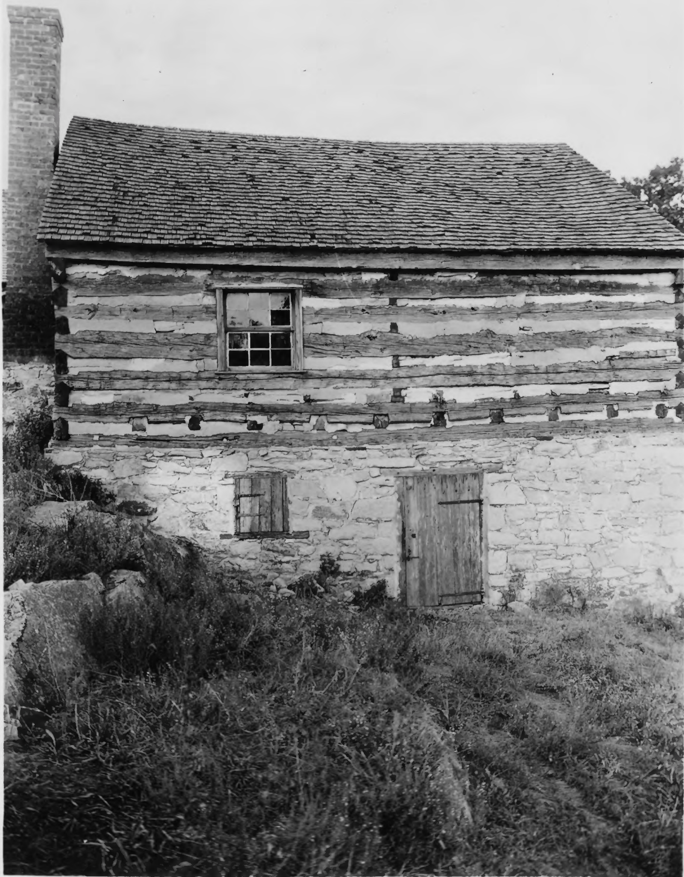
Side of Blacksmith Shop looking toward the House. The Door and Window in Stone Foundation were straightened and repaired in September 1938.
