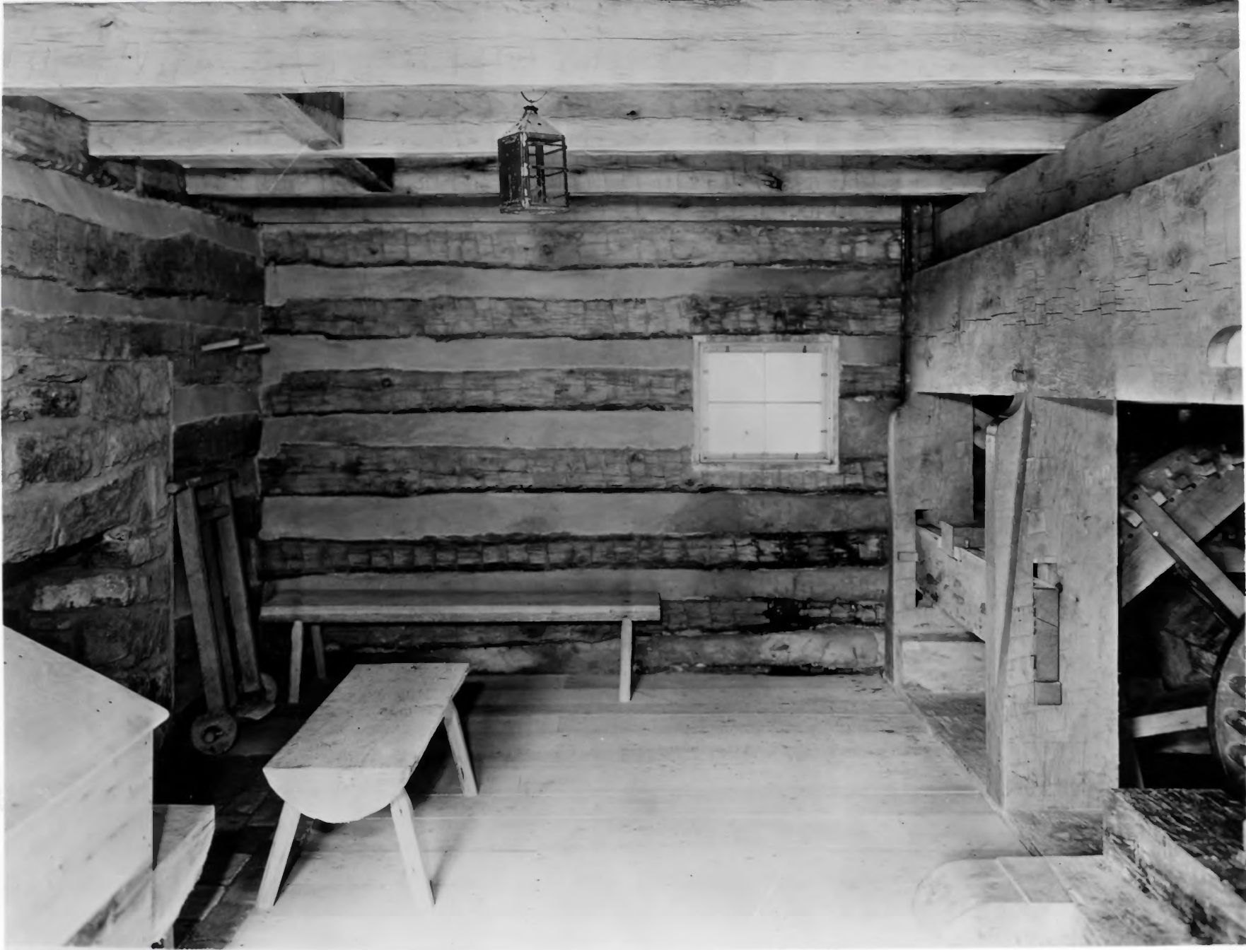
View of Interior of the Mill Building. Part of First Floor. Note Bran Bin on left and Mill Machinery on the right.
