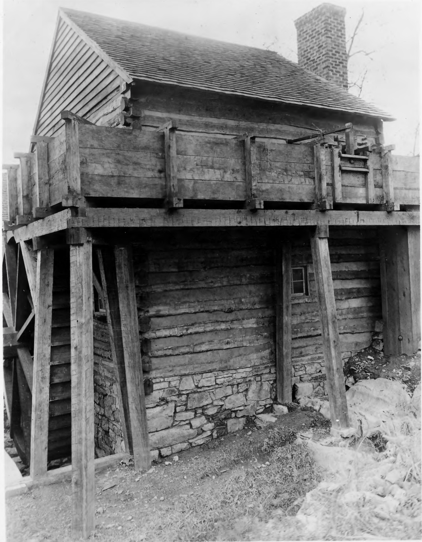
Side View of Mill showing Race. Note Spillway Gates and Levers in side of Race which control water level in Race at this point, also Water Wheel at end of Mill
