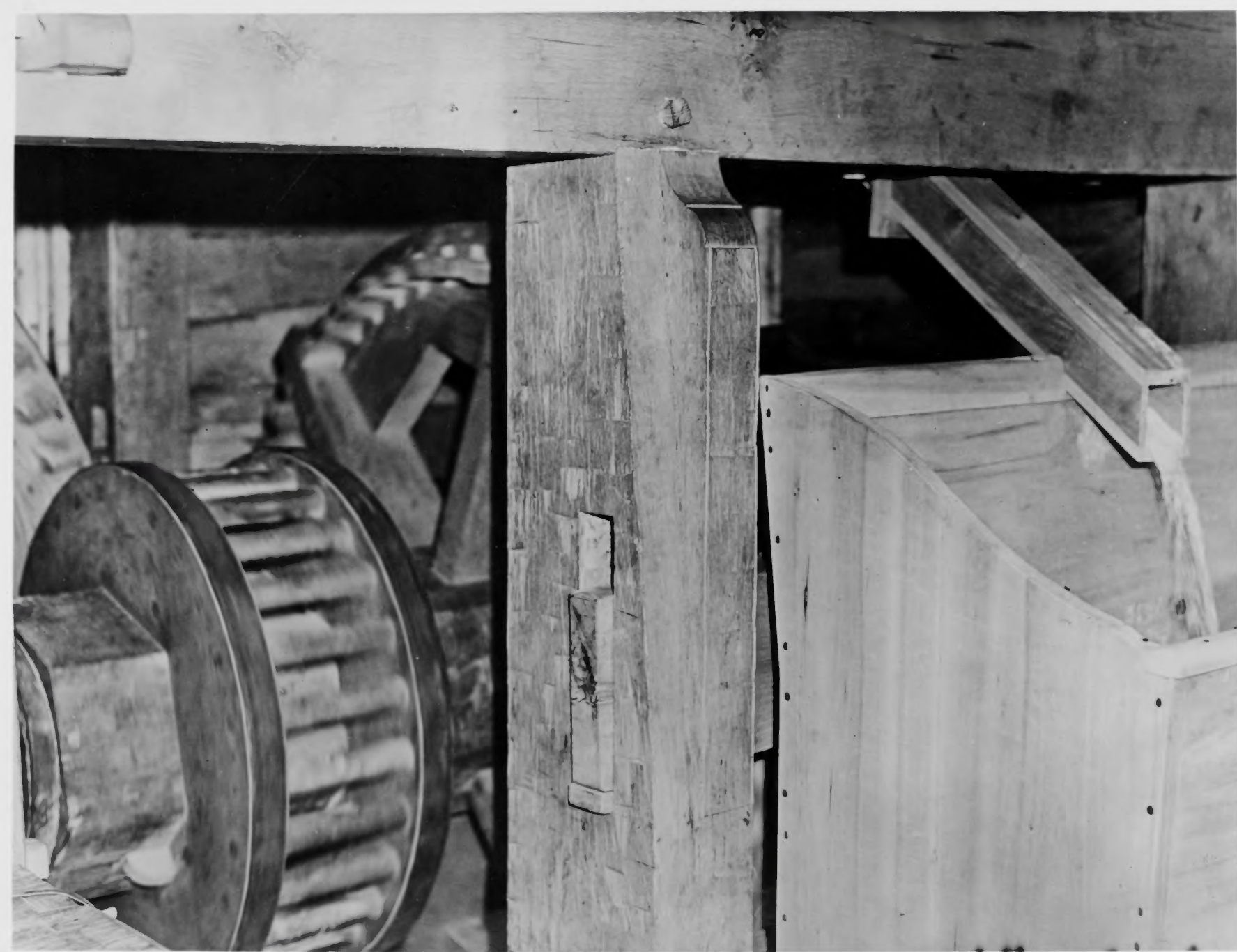
View of First Floor of Mill Building.
