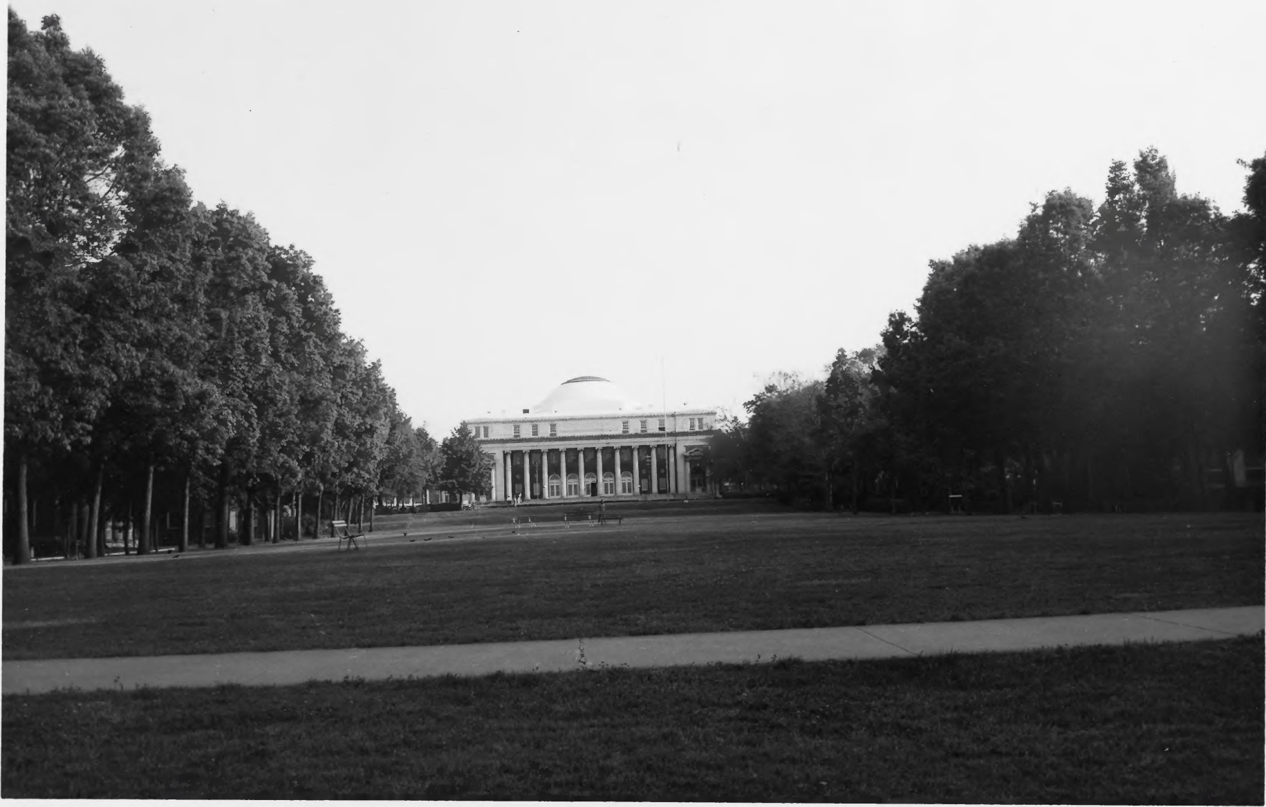
Social and Religious Building, Main quadrangle, George Peabody College for Teachers, Nashville, Tennessee
