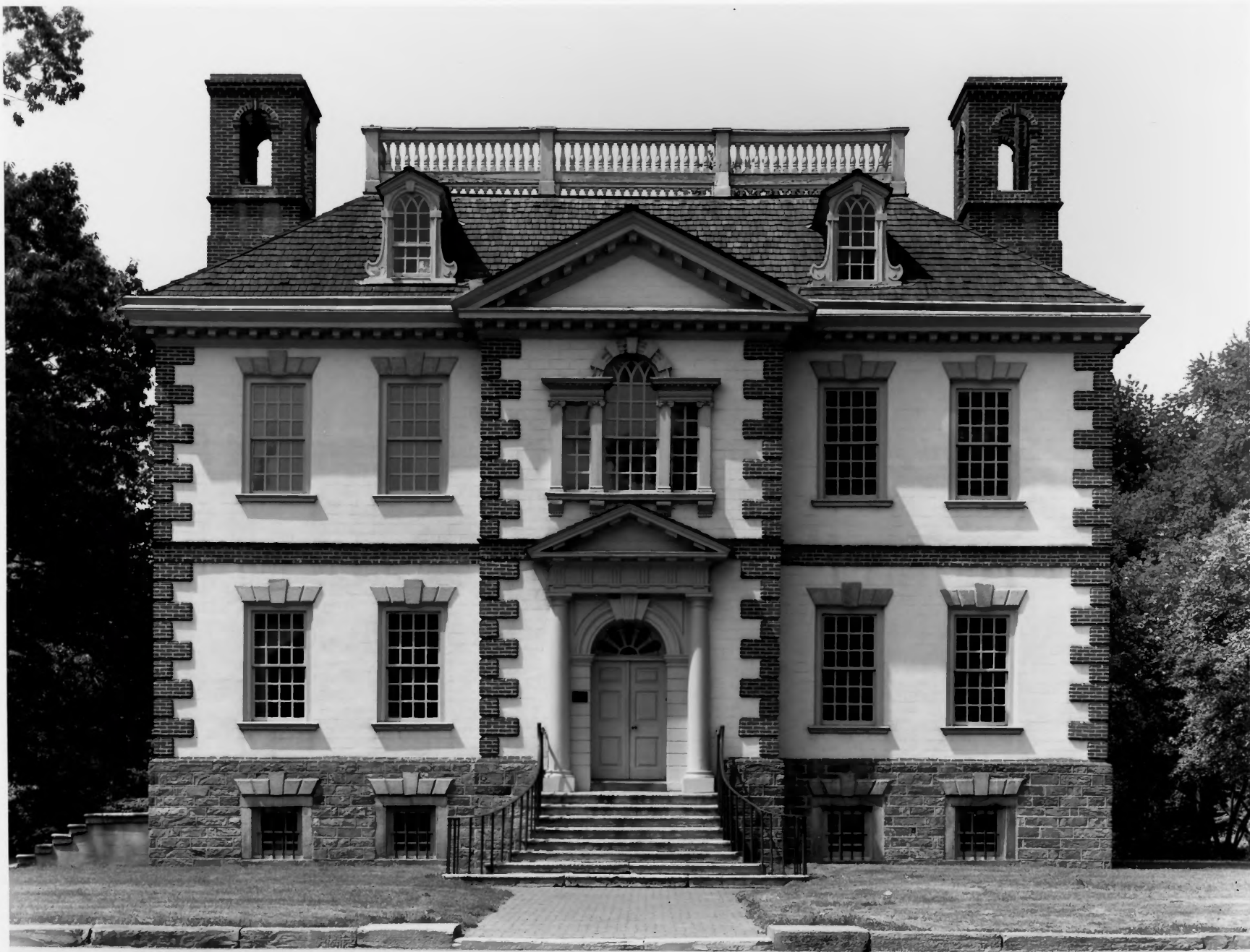
Main building Mt. Pleasant Site
