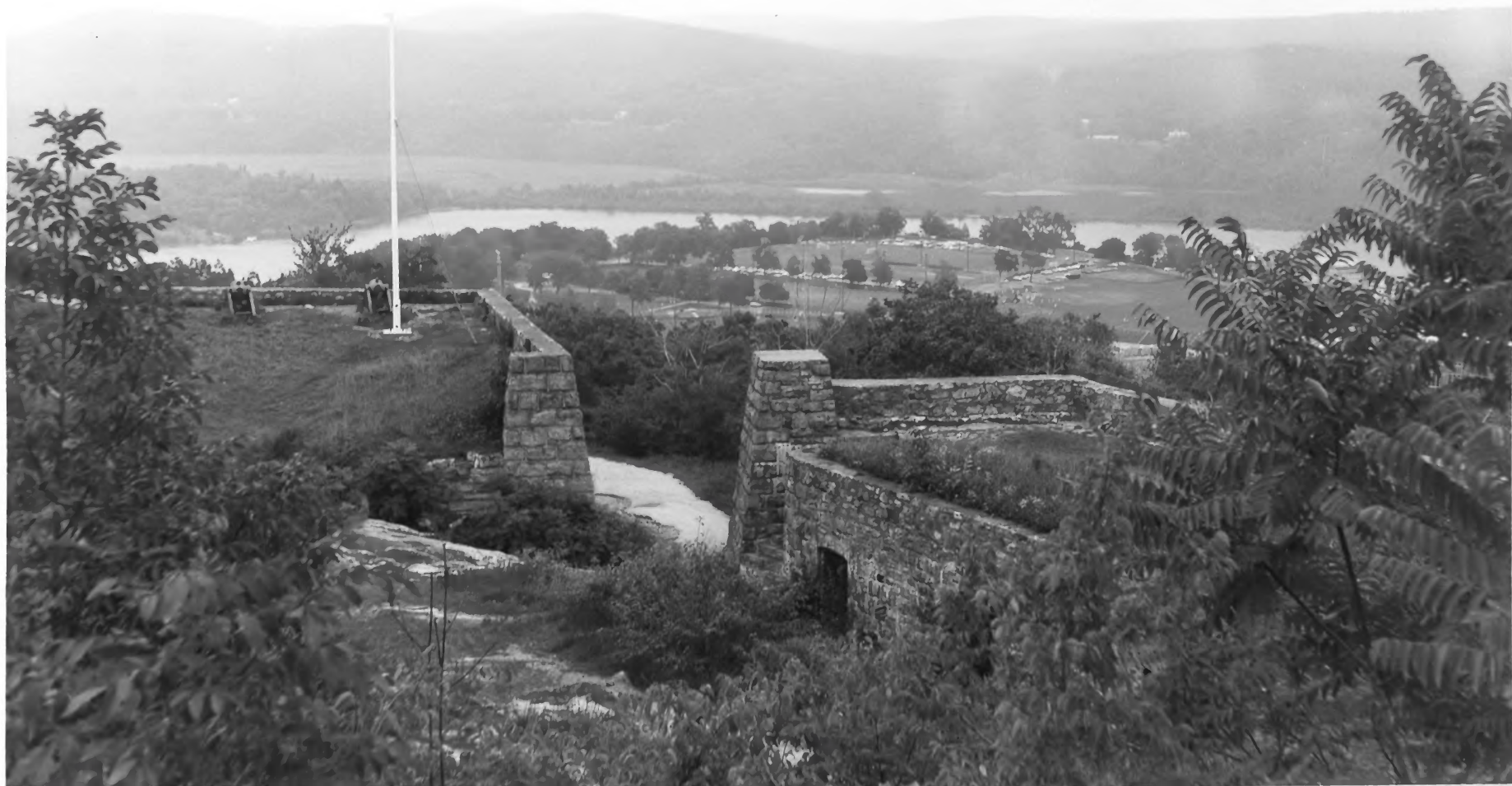
Fort Putnam (Reconstructed), looking east. West Point, New York.
