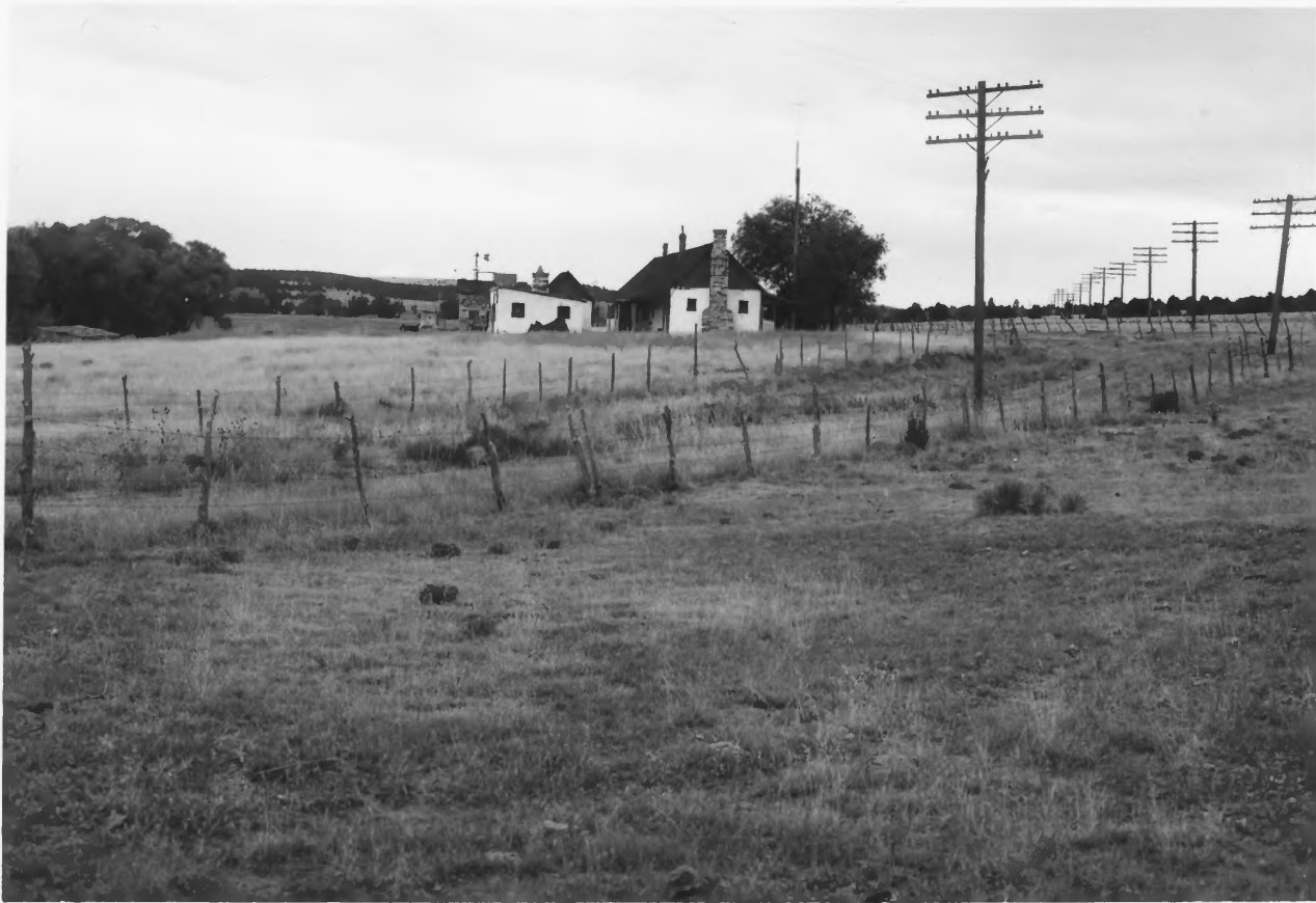
Sapello Stage Station from northeast, at original junction of Mountain and Cimarron Branches. (NPS photo by W. Brown, Oct. 1962; negative in Southwest Regional Office).
