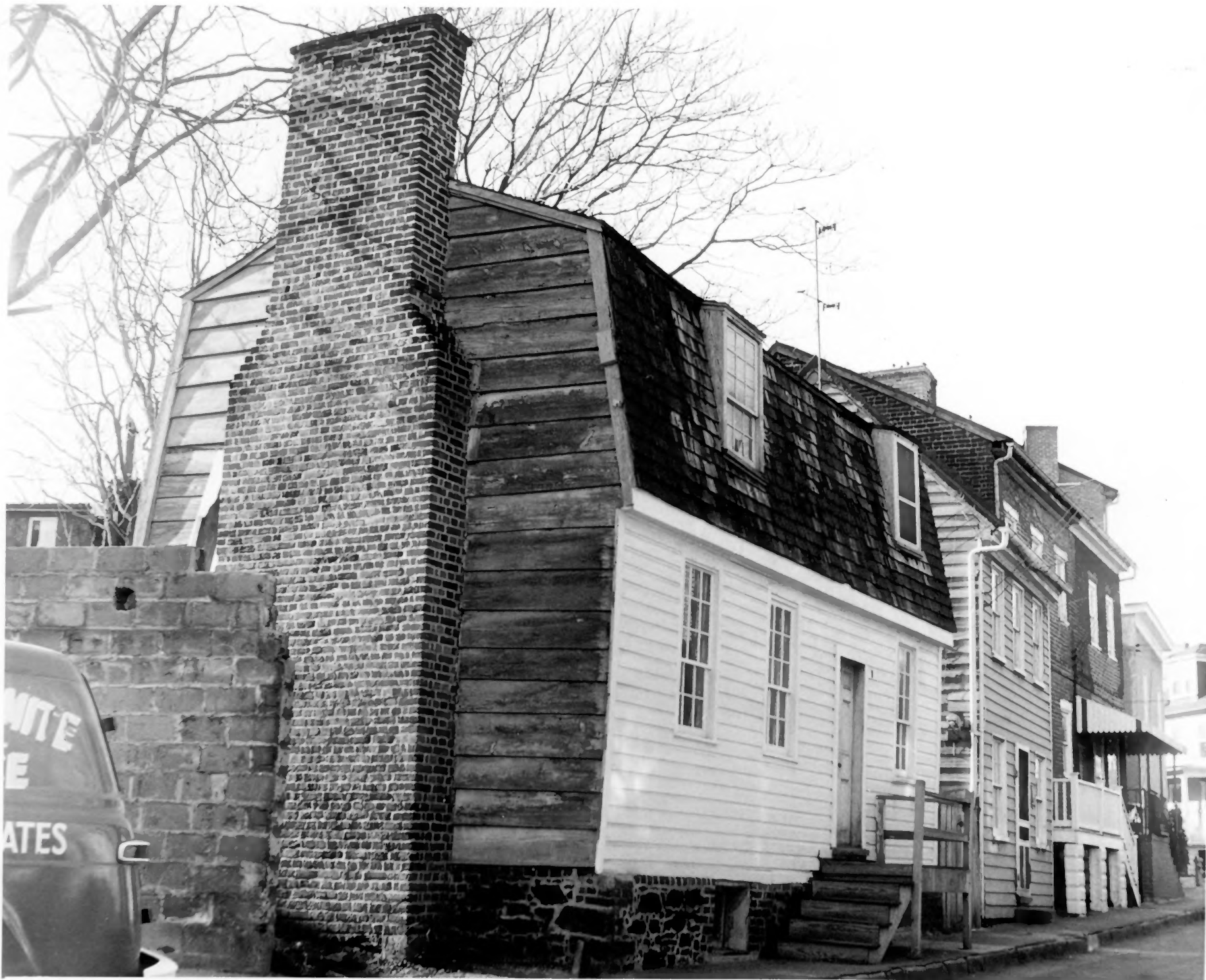
The Christopher-Hohne-Holland House, (in foreground), 45 Fleet Street, Annapolis, Maryland (NPS photo, 1964)
