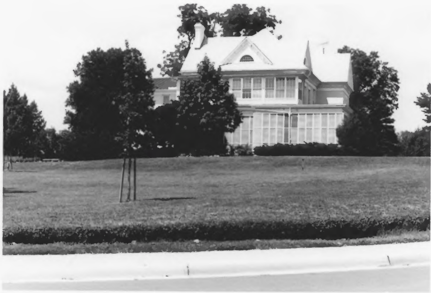
Commanding General's House. Building # 1 was built in 1861 to house the Commanding Officer, Fort Leavenworth Arsenal. Additions and modifications have been made through the years.
