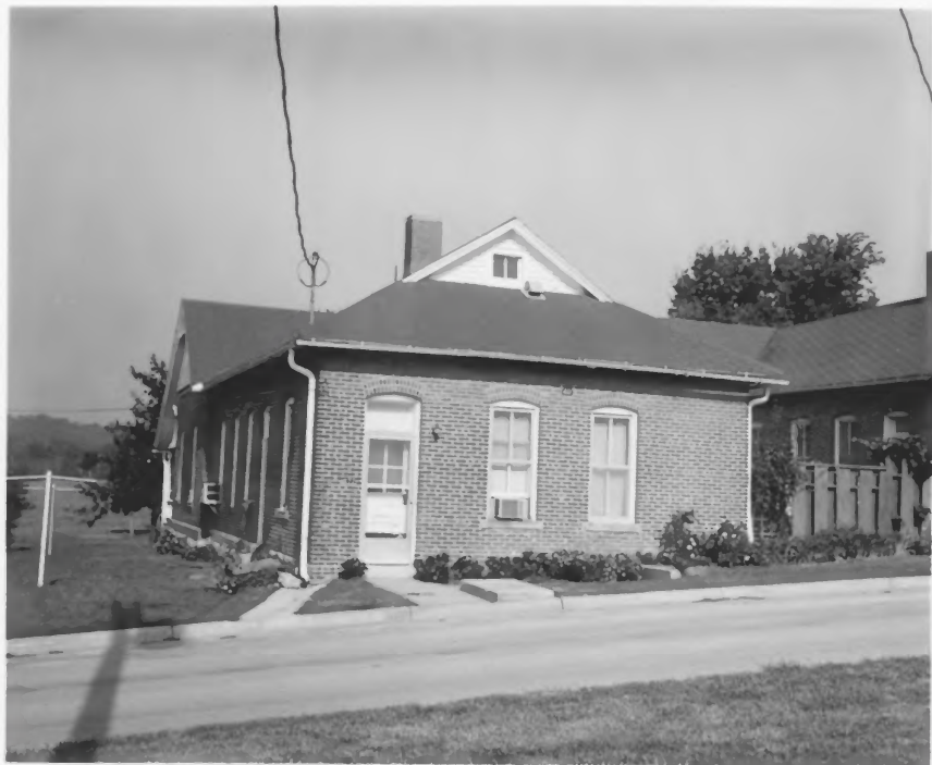
Building 40 620 Thomas Ave. Rear view looking Northwest July 1976
