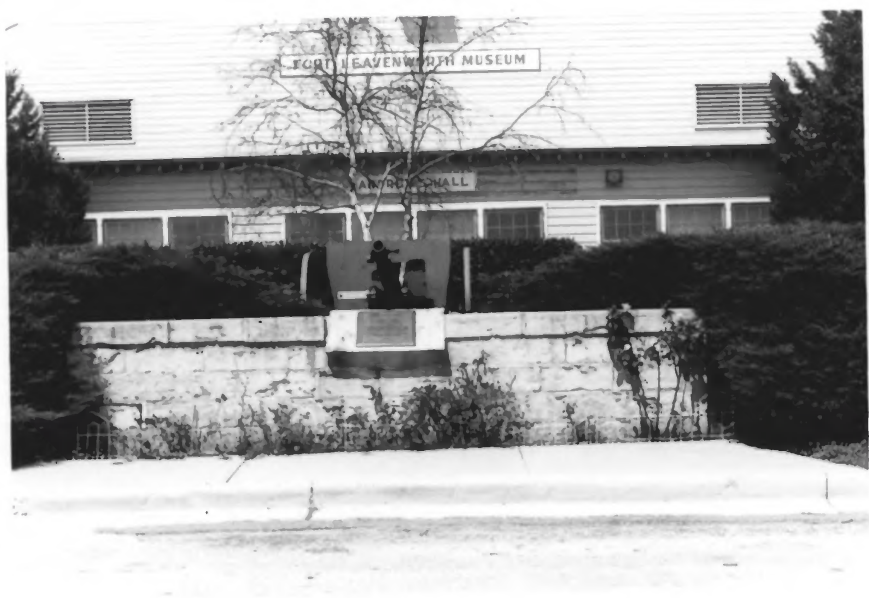
Fort Leavenworth Museum, a World War II vintage structure (not located within the Landmark District boundary) houses the interpretive and educational exhibits for Post visitors. Note location of the Landmark Plaque.
