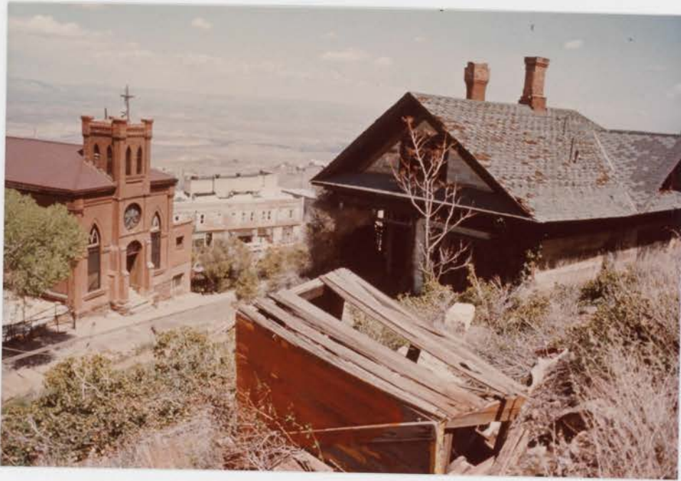
EPISCOPAL CHURCH UNDER RESTORATION, TO BE HOME OF JEROME HIST. SOCIETY
