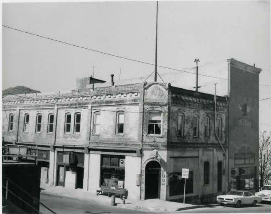
Hotel Conner, looking North
