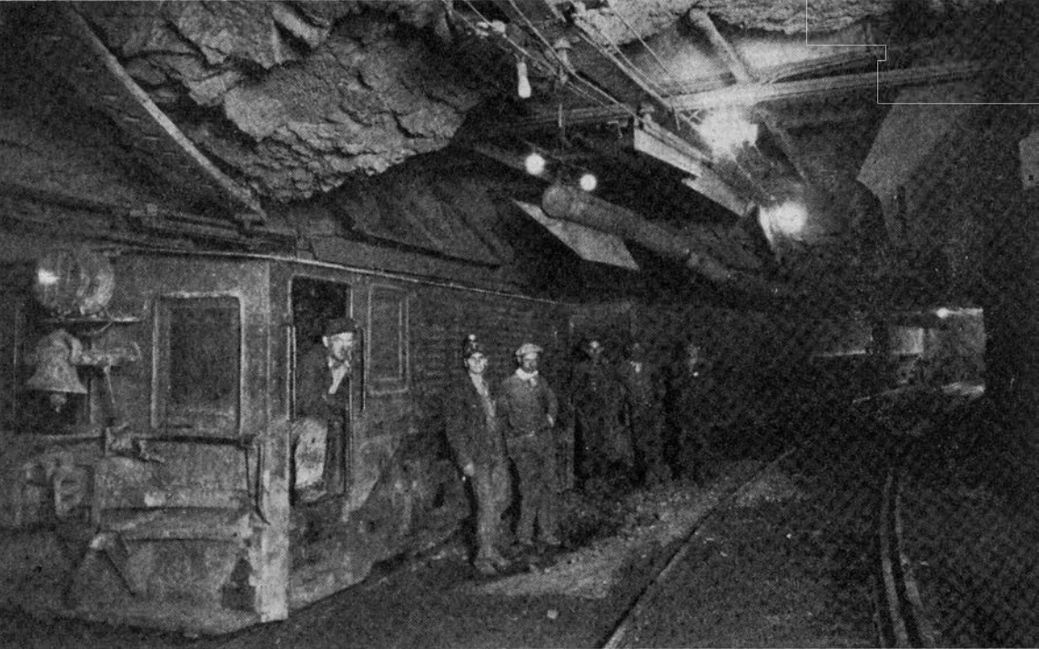
Electric train and train crew in the Hopewell haulage tunnel.
