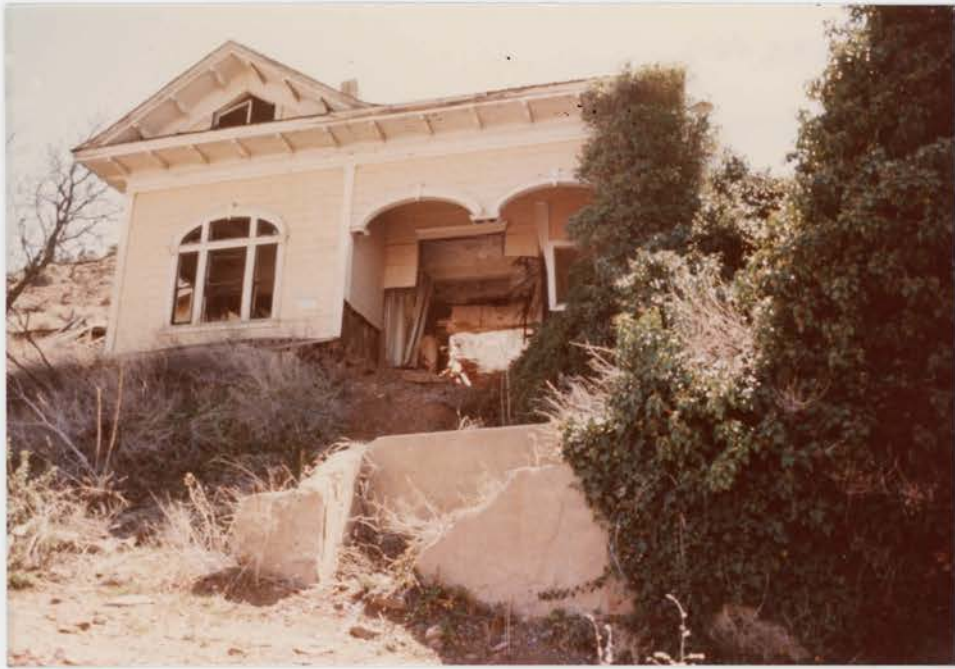
Decaying Victorian House
