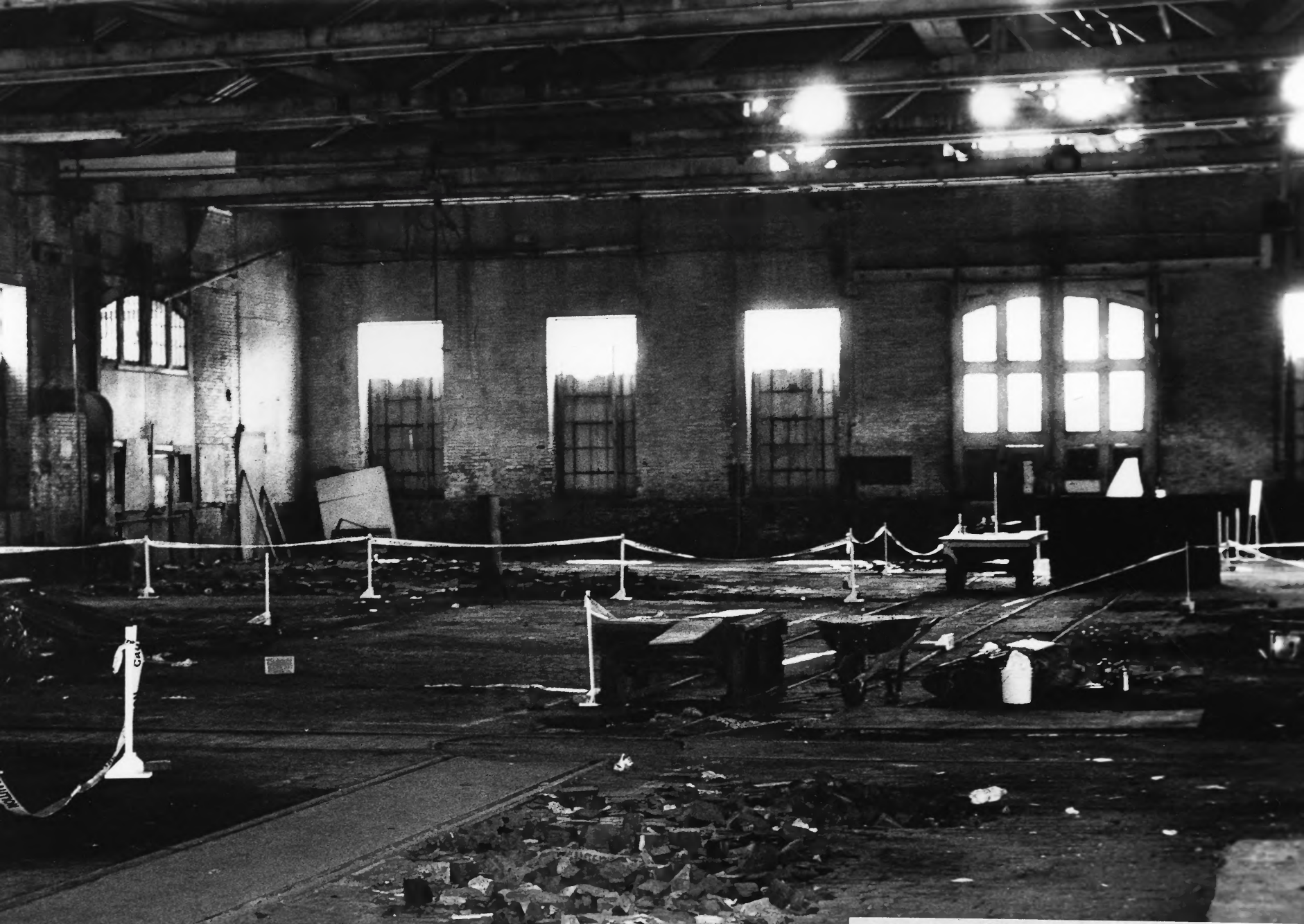
Photograph #12 B&O RAILROAD MARTINSBURG SHOPS Martinsburg, WV Interior of Car Shop, looking west. Michael Caplinger, IHTIA, August 2001
