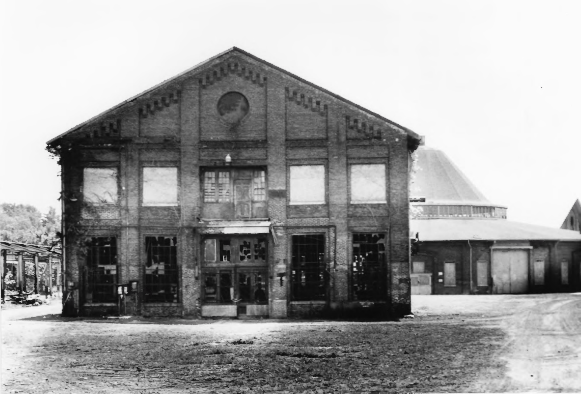
Photograph #2 B&O RAILROAD MARTINSBURG SHOPS Martinsburg, WV North facade of Machine/Woodworking Shop, looking south. Michael Caplinger, IHTIA, August 2001
