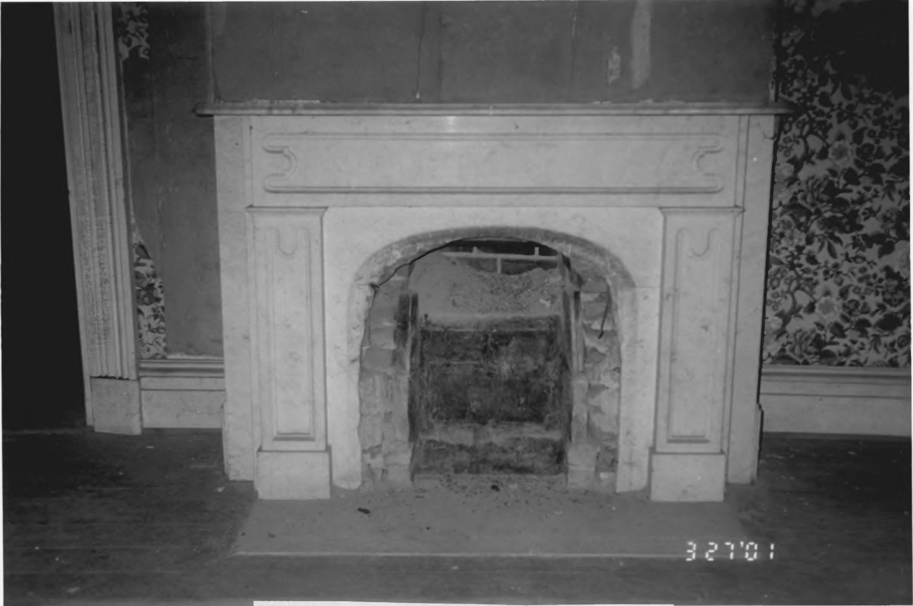
DR. OLIVER BRONSON HOUSE AND ESTATE Hudson, New York Marble mantelpiece, first-story southwest room of 1849 addition Photo by Peter Shaver and Bill Krattinger, 2001
