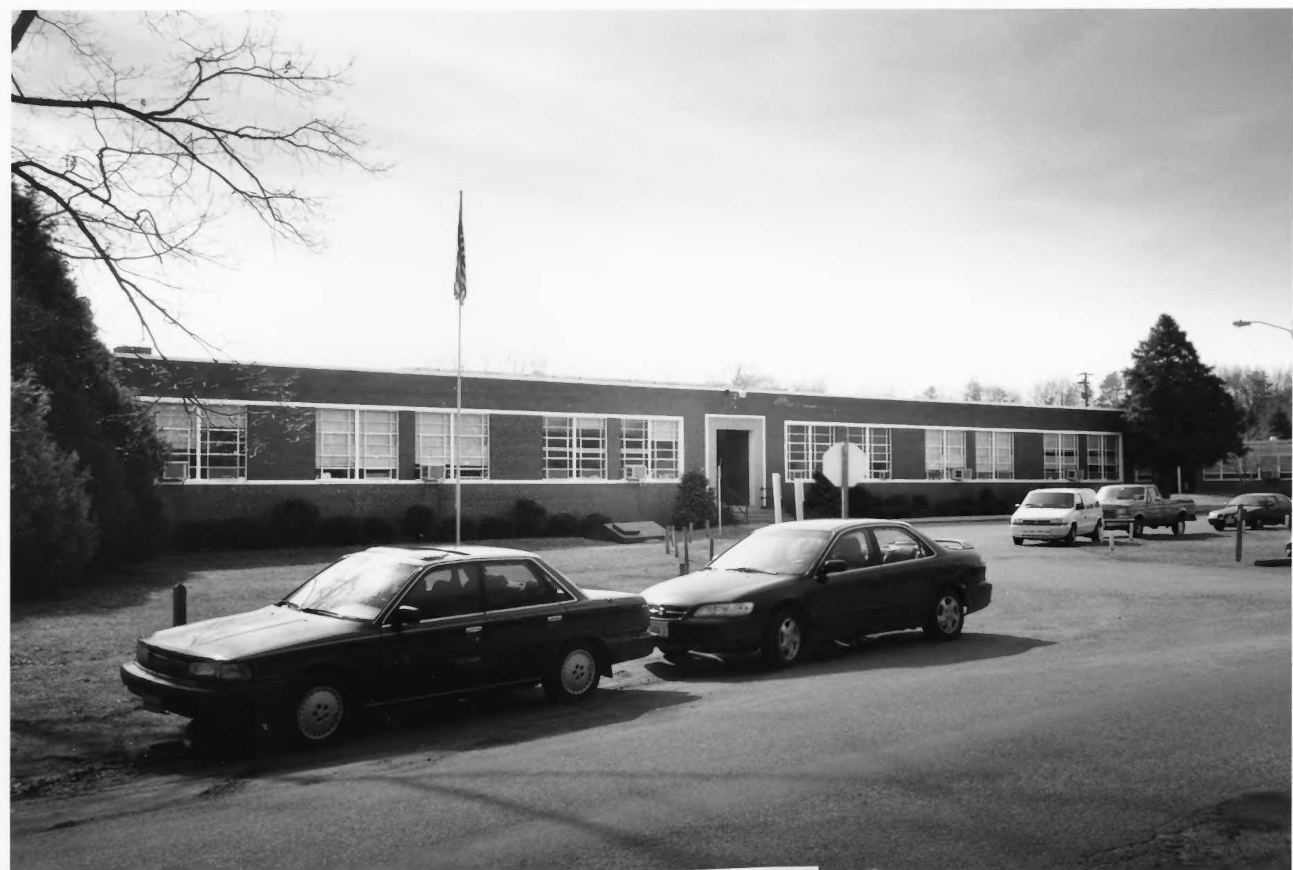
Figure 5. George W. Watkins School 1950 Building, Front Elevation
