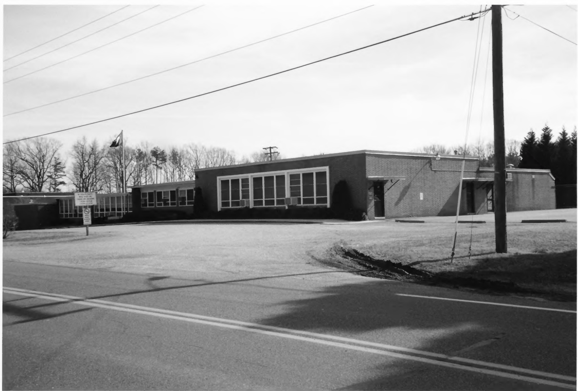
Figure 6. George W. Watkins School 1960 Building, Front and West Elevations
