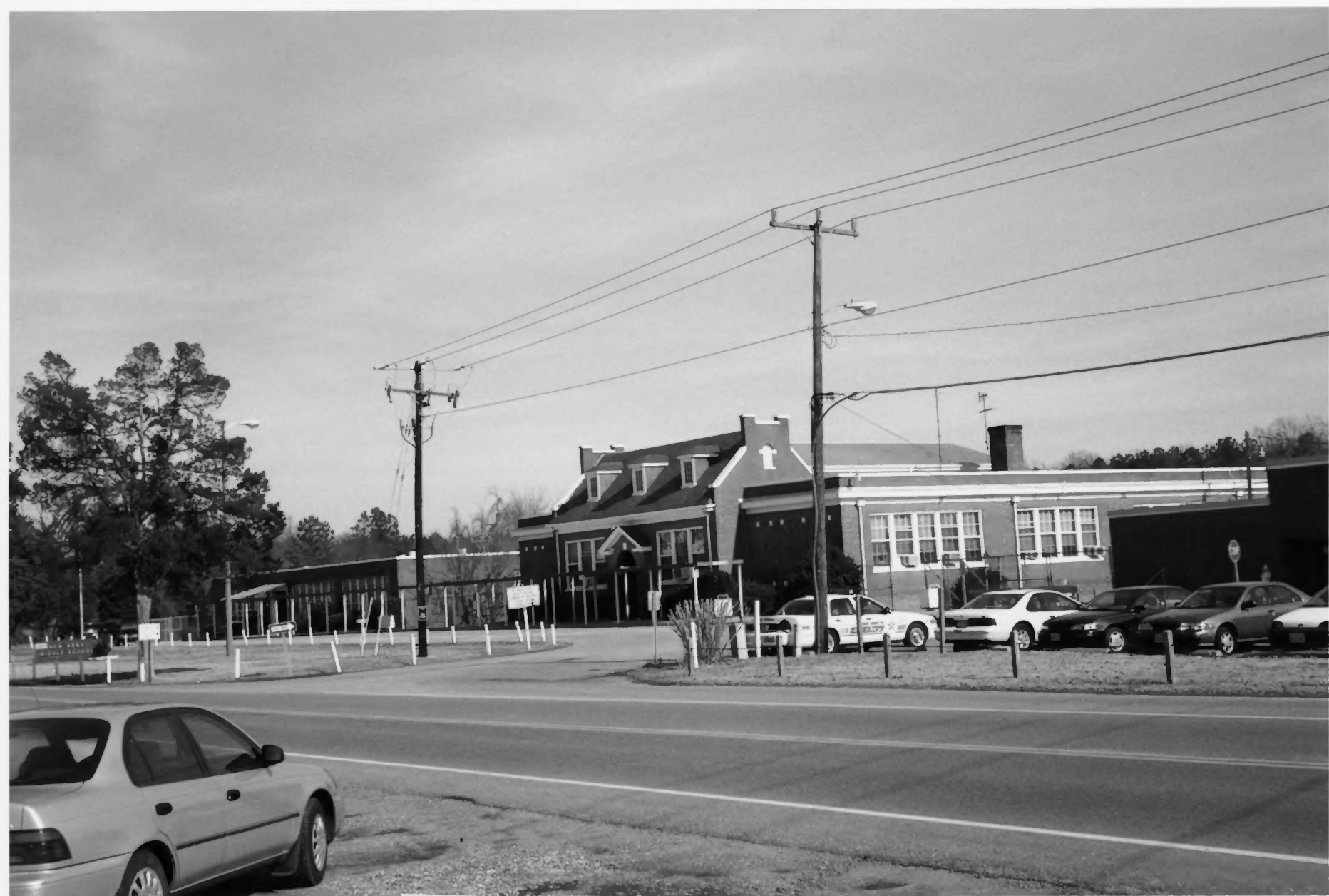
Figure 1. New Kent School Front and West Elevations
