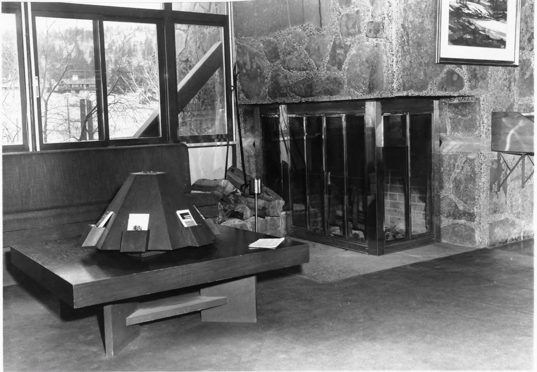
Figure 8 Rocky Mountain National Park Administration Building Larimer County, Colorado Interior detail, 1982
