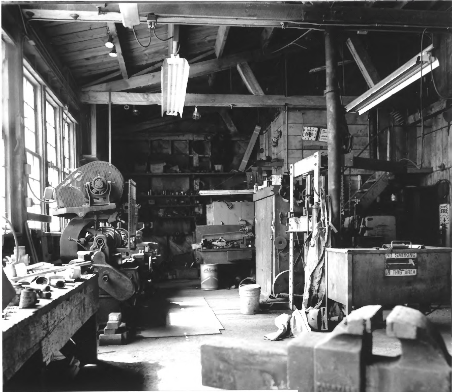
Photograph #32 Shenandoah-Dives Mill Silverton Vicinity, San Juan County, Colorado Interior of Mill Workshop Frederick Athearn, Historian, San Juan County Historical Society , September 1995
