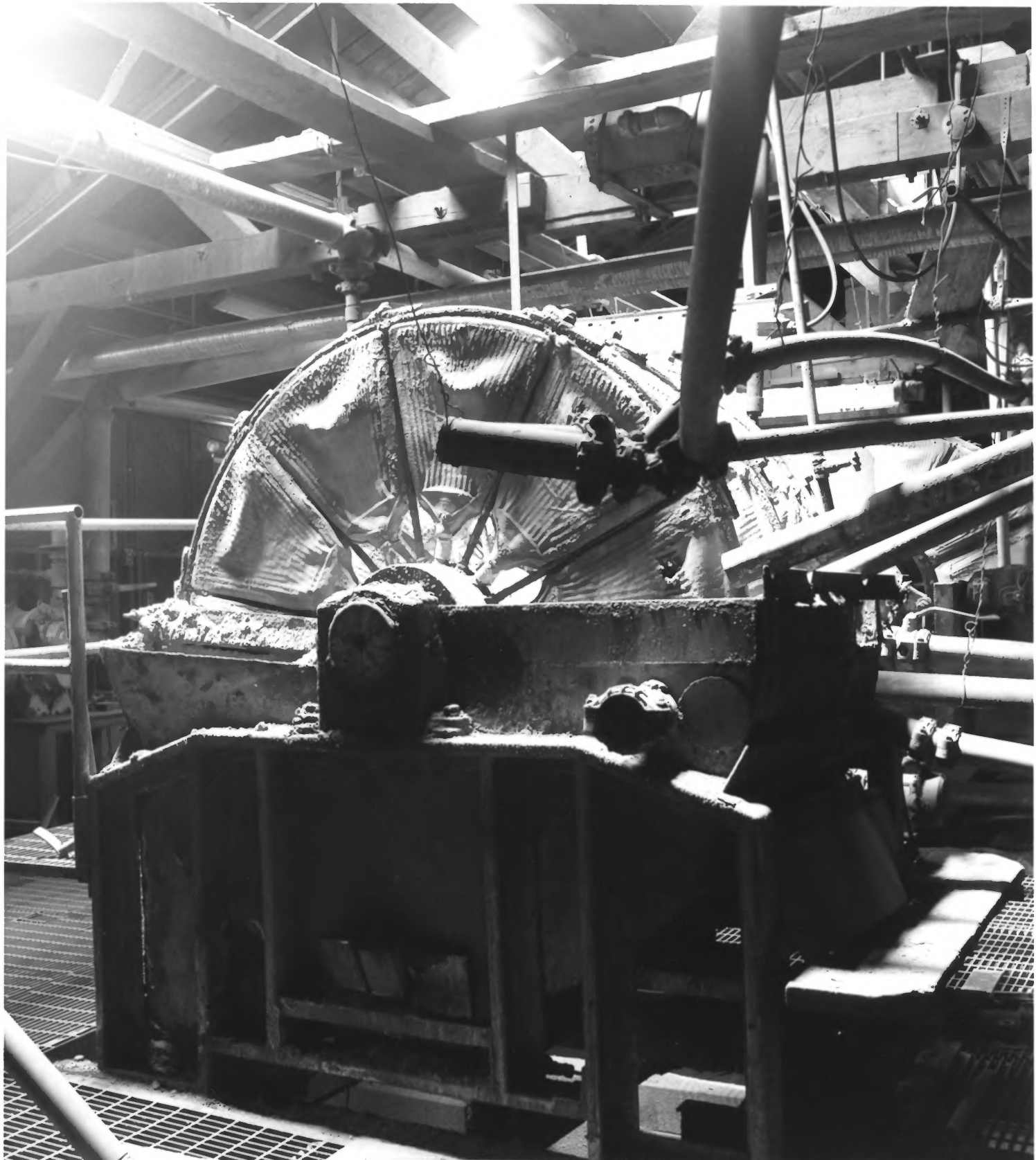
Photograph #31 Shenandoah-Dives Mill Silverton Vicinity, San Juan County, Colorado Canvas Wheel Filter (#32 & 33 on Flow Chart) Silver Rich Images (John Matsko), Olathe, Kansas, August 1998
