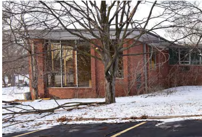
Figure 24: Resource 1, Block H, southeast corner. Source: Brad Finch, F-Stop Photography, March 2015.
