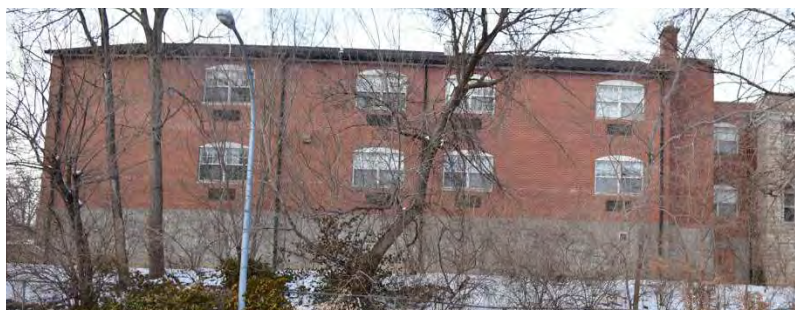
Figure 31: Resource 1, Block K, south elevation. Source: Brad Finch, F-Stop Photography, March 2015.
