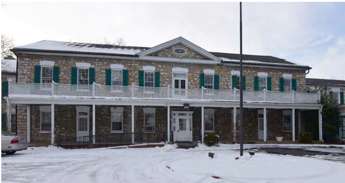
Figure 7: Resource 1, Block A, east elevation. Source: Brad Finch, F-Stop Photography, March 2015.
