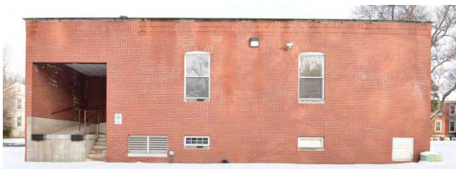
Figure 28: Resource 1, Block J, west elevation. Source: Brad Finch, F-Stop Photography, March 2015.
