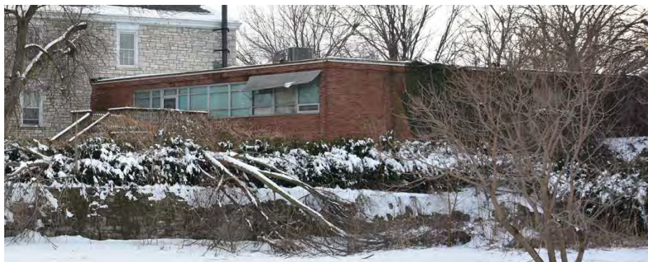
Figure 18: Resource 1, Block F, east elevation. Source: Brad Finch, F-Stop Photography , March 2015.
