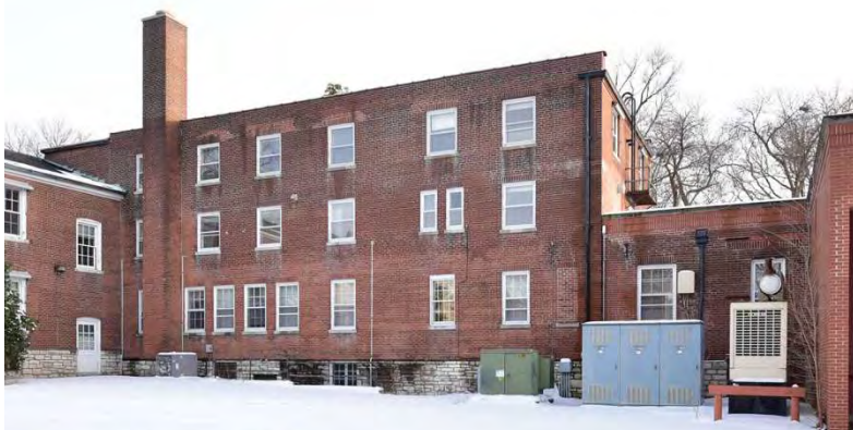
Figure 11: Resource 1, Block C, north elevation. Source: Brad Finch, F-Stop Photography, March 2015.
