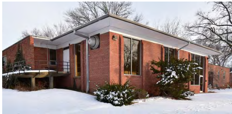
Figure 25: Resource 1, Block H, northwest corner. Source: Brad Finch, F-Stop Photography, March 2015.
