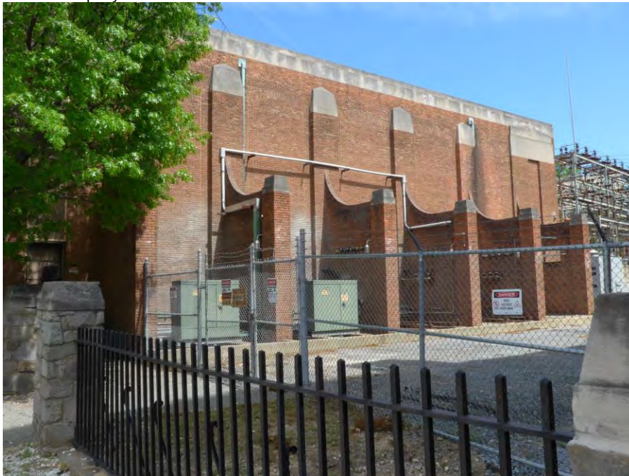
Pepco Substation No. 25
