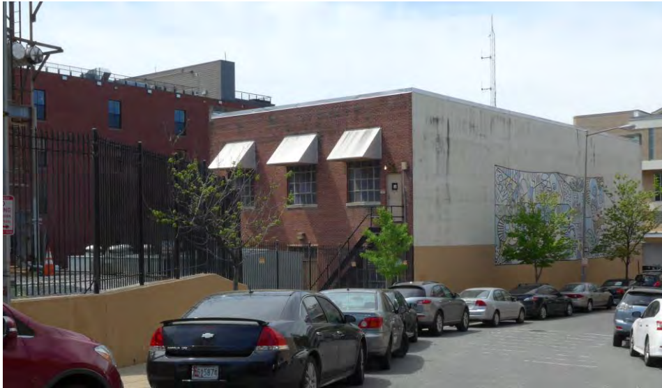
Pepco Substation No. 25 General View looking southwest 4/8
