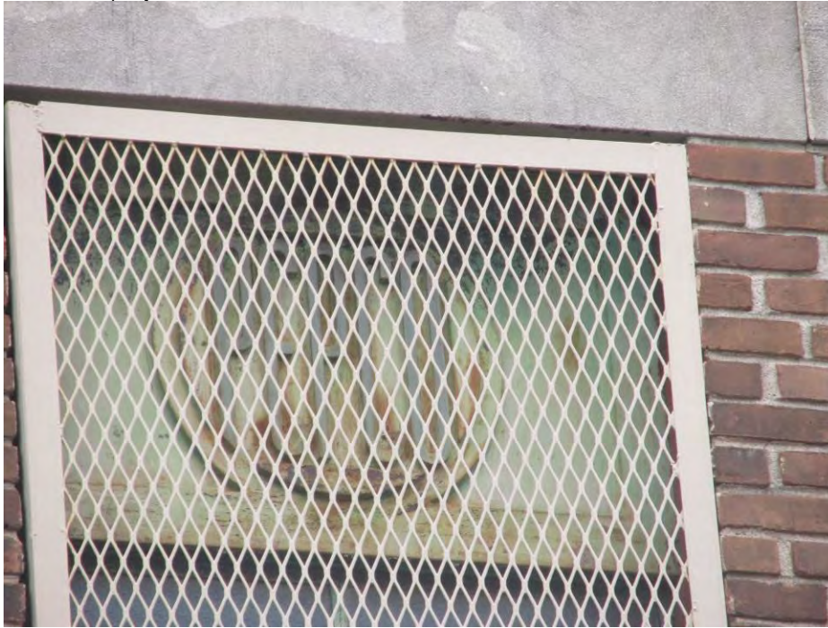
Pepco Substation No. 25 Detail of Iron Spandrel Above Champlain Street Windows 6/8
