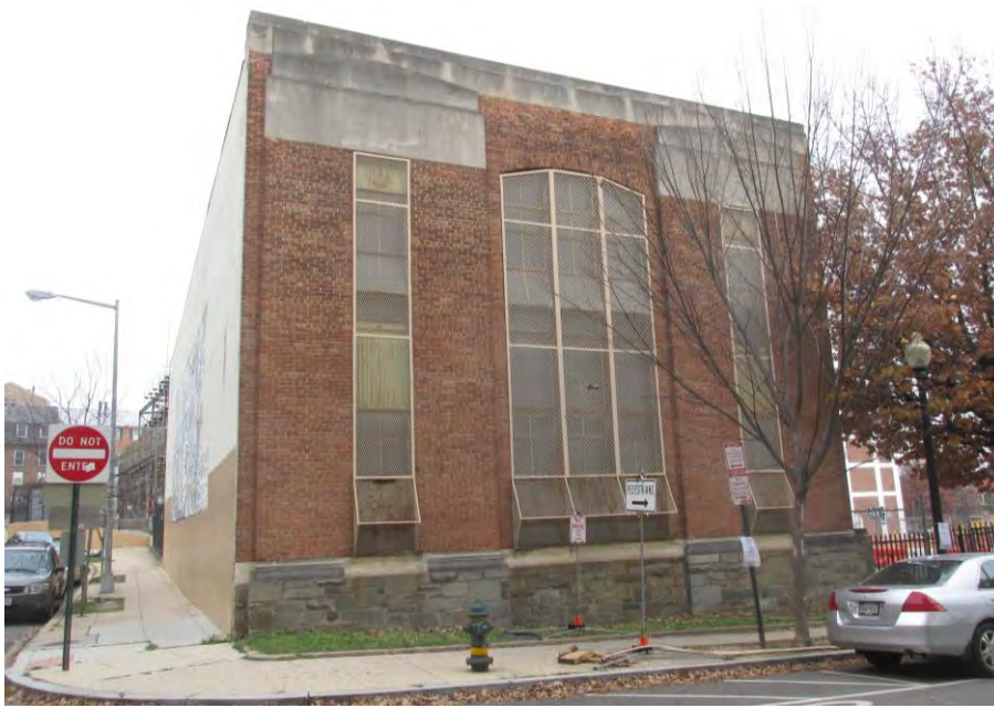
Pepco Substation No. 25 General View looking east southeast showing Champlain Street façade 1/8
