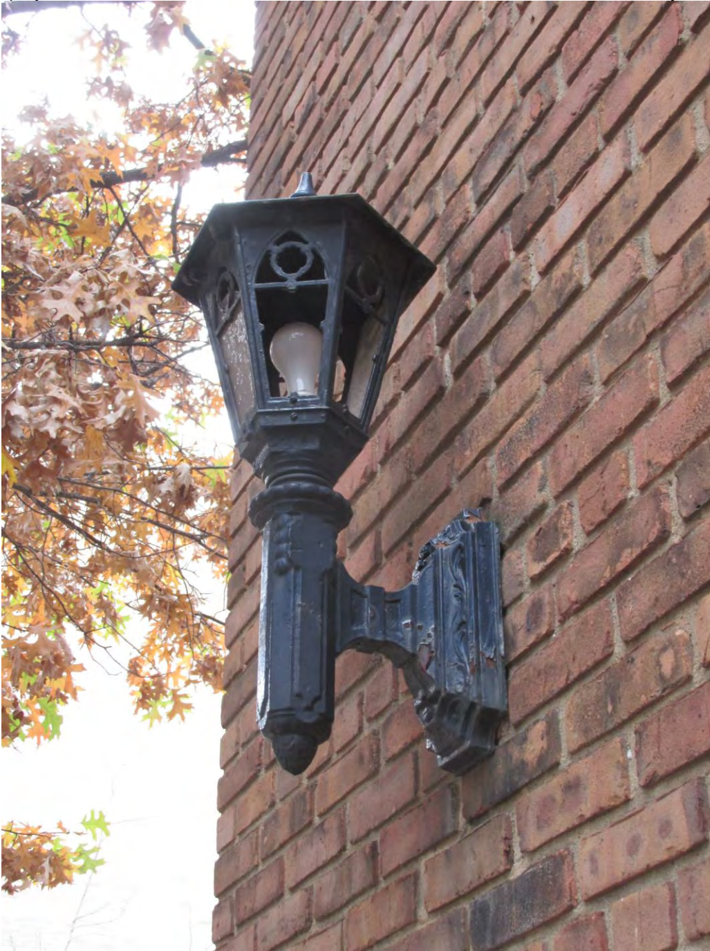
Pepco Substation No. 25 Detail of Outdoor Entrance Light 7/8
