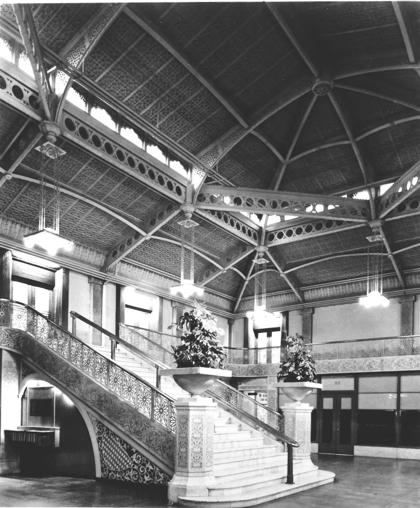
The Rookery, Chicago, Illinois Interior Lobby
