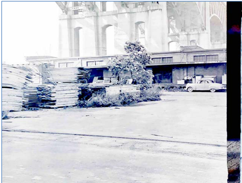
Figure 22b. Consolidated Fruit Auction Building, section of east elevation at Central Avenue, 1955. Photographic negative converted to positive. Source: Cuyahoga County Archives, Cuyahoga County Engineers records, Lorain-Carnegie Bridge files.
