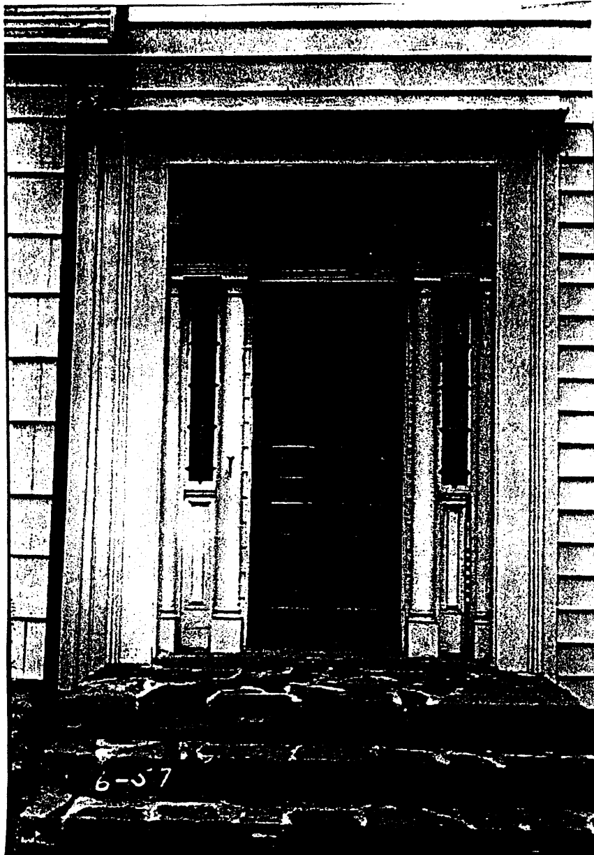
Figure 11. By the time the HABS team visited in 1936, the porch had been removed and stone steps built in front of the east wing. The ornamental lead in the sidelights and transom still was in excellent condition.
