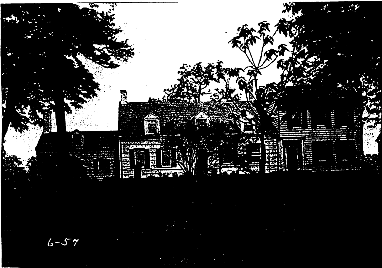
Figure 9. By the time the Historic American Buildings Survey photographed the Staats House in 1936, the Riddells had removed the shed-roofed dormers, replacing them with the gable-roofed dormers that still survive.
