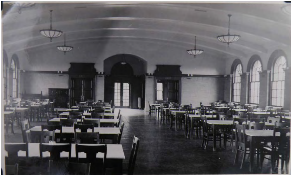
Figure 25: Interior view of main dining room, 1920s (Chicago History Museum)
