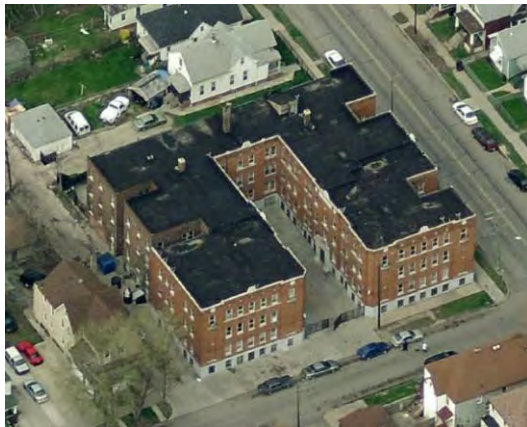
Figure 23: The relatively unusual central courtyard plus light courts arrangement of 2215 Lansing Street, from Bing Maps.
