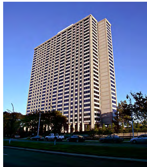
Figure 58: 1300 Lafayette East, from the Lafayette East Cooperative.
