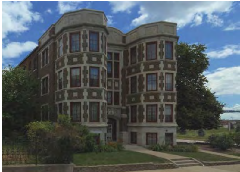
Figure 18: The paired bay front Savannah at 250 West Grand Boulevard, from Google Streetview.
