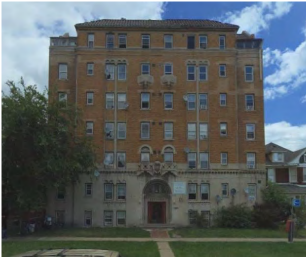
Figure 38: The Barbara Apartments at 512 West Grand Boulevard, from Bing Streetside Maps.
