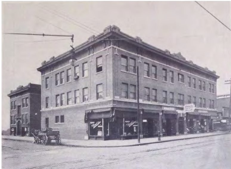
Figure 16: A typical commercial apartment building from the 1920s, at Hastings and Adelaide (no longer extant), from D/Apartments-General, Burton Historical Collection, Detroit Public Library.
