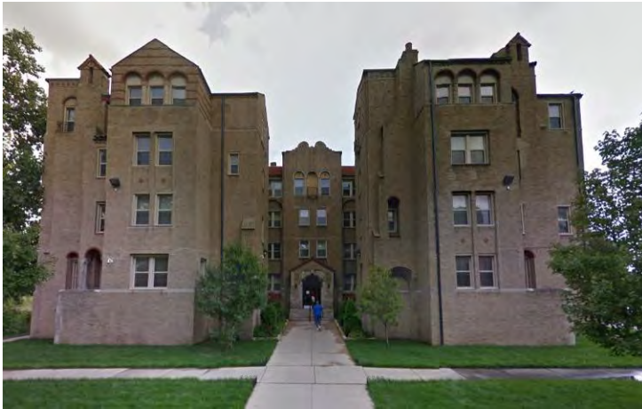
Figure 45: Andorra Apartments, 2725 Boston, from Google Streetview.
