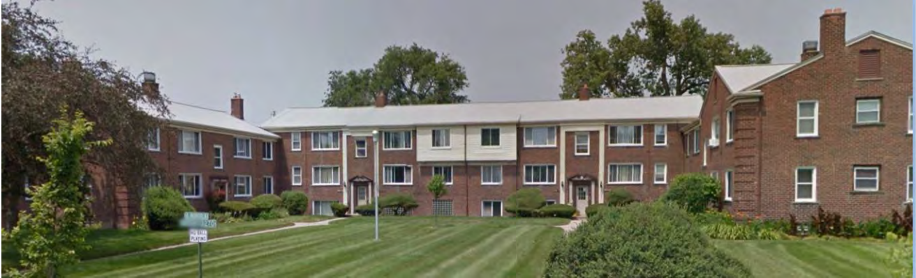
Figure 55: Blackstone Cooperative Apartments at Eight Mile Road and Schaefer, from Google Streetview.
