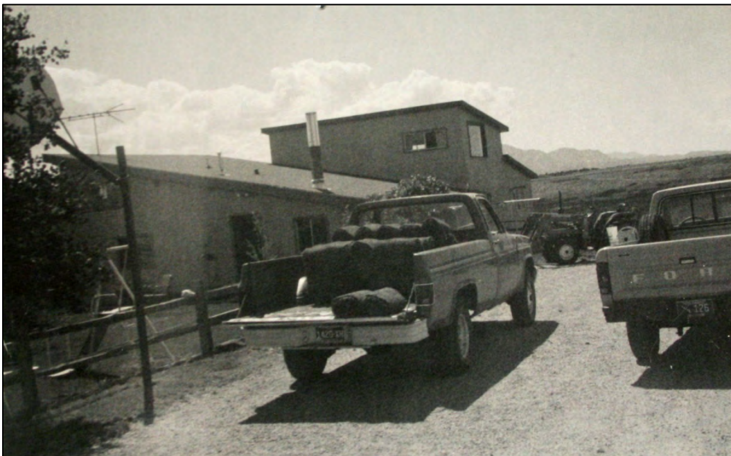
Figure 5. The former bunkhouse took on a new look after Bryce and Suzy Kelly's remodeling and expansion, as shown in this ca. 1970s-80s assessor card photograph (view southeast) (Resource 12). Courtesy of Chaffee County Assessor, old real property appraisal card, Salida, Colorado.
