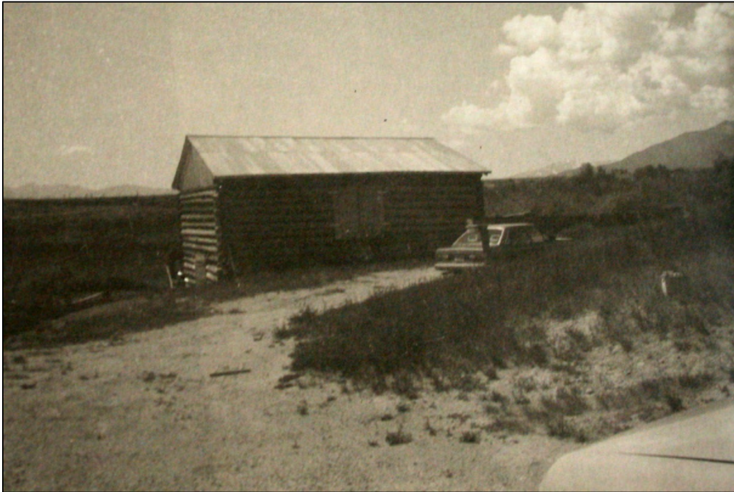
Figure 6. The bank barn (Resource 10) at the south end of the headquarters had a somewhat steeper roofline, as shown in this ca. 1970s-80s assessor card photograph (view south-southwest). After storm damage the roof was rebuilt with its current, shallower slope. Courtesy of Chaffee County Assessor, old real property appraisal card, Salida, Colorado.
