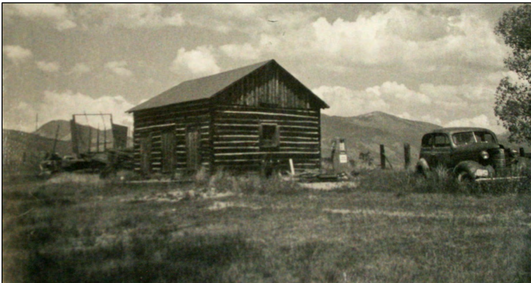
Figure 3. The granary (Resource 6) is shown in this ca. 1970s-80s assessor card photograph (view west-northwest). Courtesy of Chaffee County Assessor, old real property appraisal card, Salida, Colorado.
