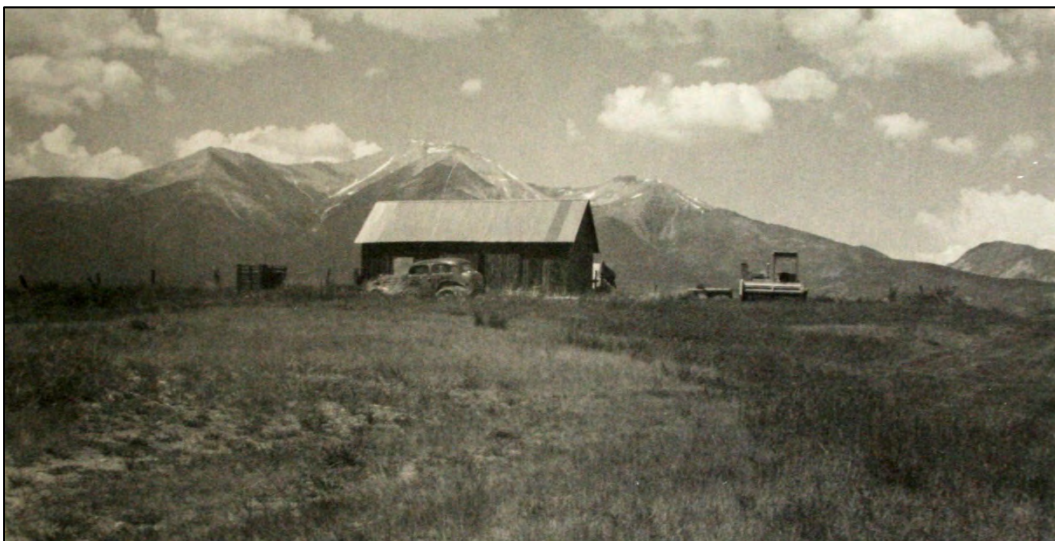
Figure 7. The blacksmith shop stood on the west edge of the headquarters until it was blown down by strong winds ca. 1996. Its concrete foundation remains. It is shown in this ca. 1970s-80s assessor card photograph (view west). Courtesy of Chaffee County Assessor, old real property appraisal card, Salida, Colorado.
