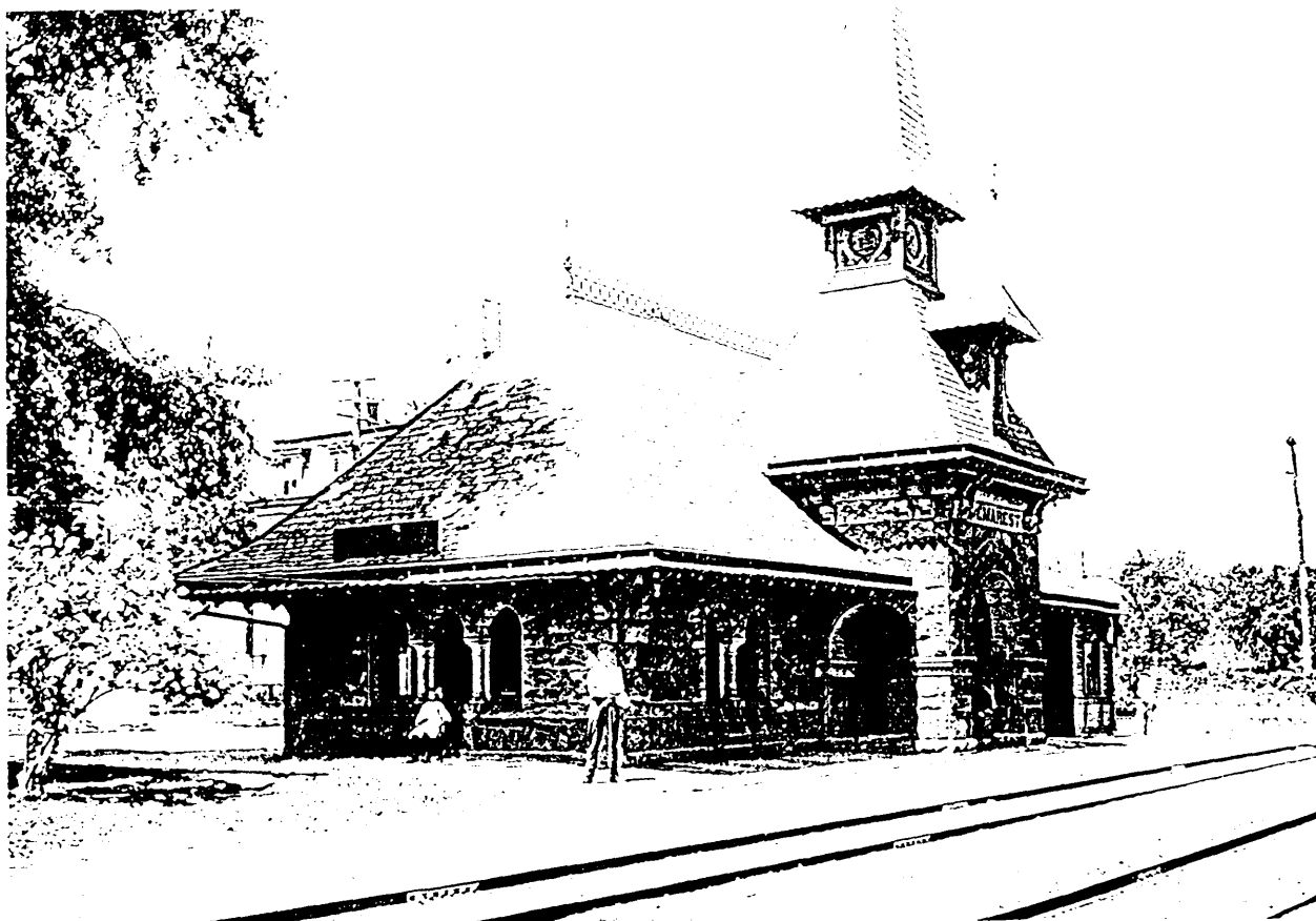
M.P. 19.2 DEMAREST was originally a flag stop on the Northern. At the time of these pictures, eighteen trains in each direction made weekday stops.
