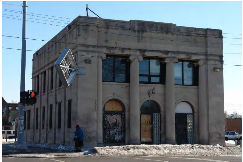
Figure 10: The Detroit Savings Bank branch at 7968 Kercheval.
