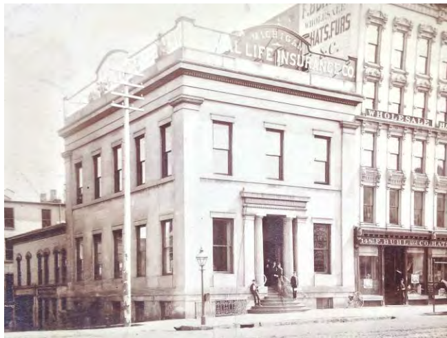
Figure 1: The Bank of Michigan’s 1836 building at Jefferson and Griswold, from the Burton Historical Collection (unknown date).
