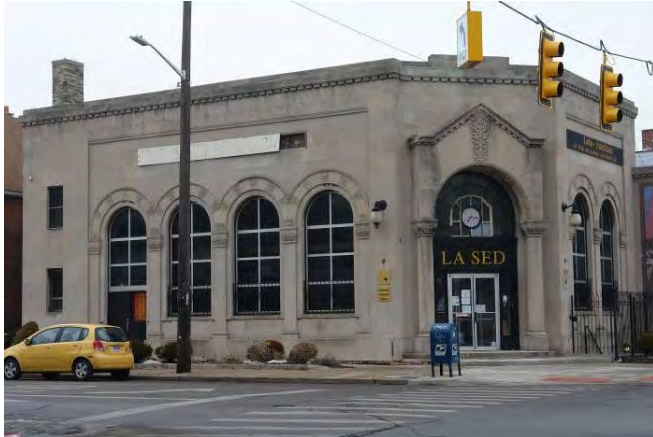
Figure 20: The Wayne County and Home Savings Bank Branch at 4138 West Vernor Highway.
