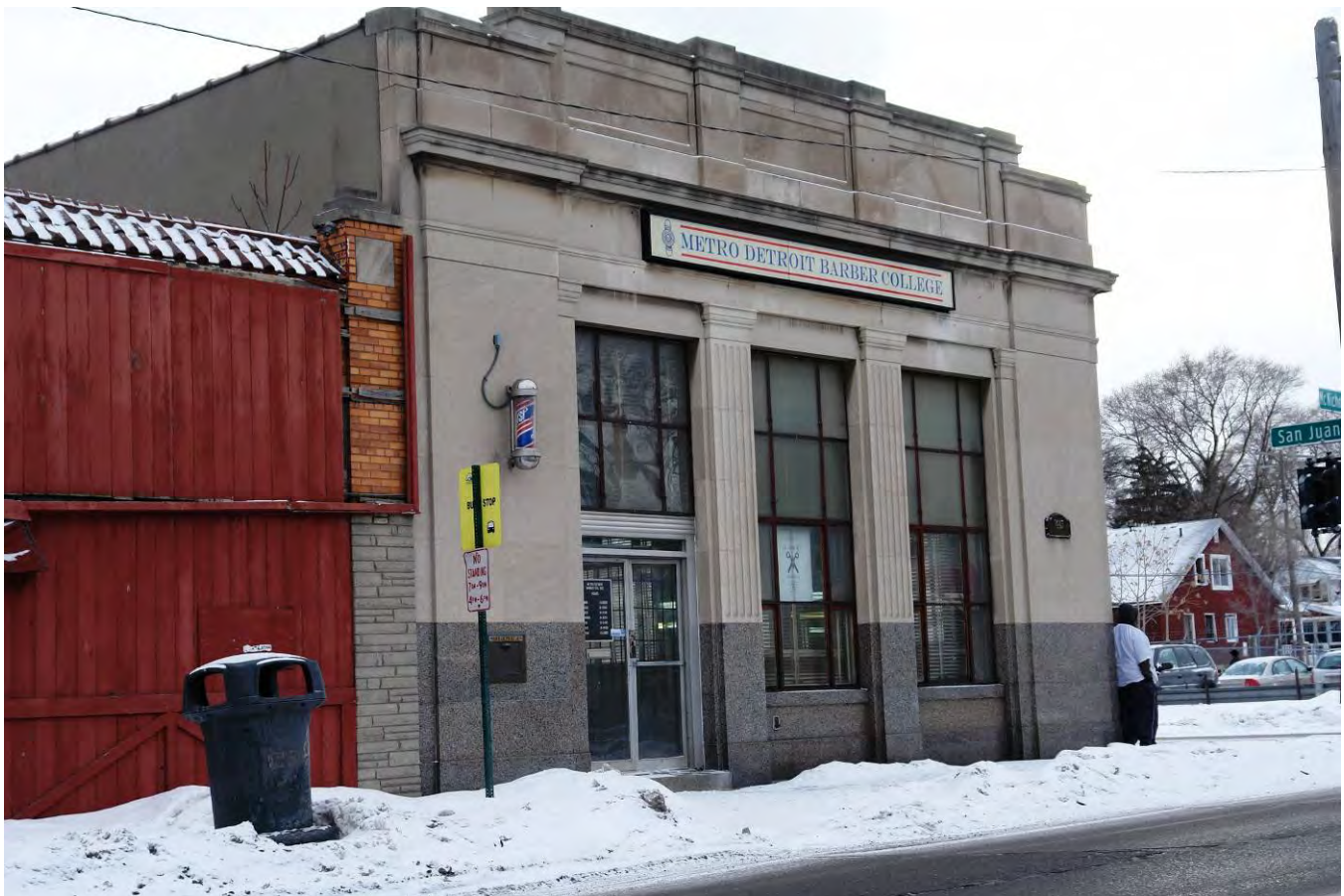
Figure 47: First National Bank branch at 7443 West McNichols.
