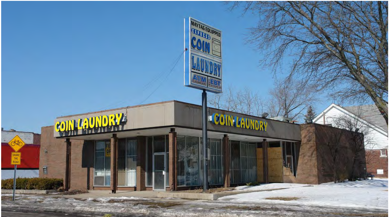
Figure 43: City Bank branch at 15541 East Warren and Somerset.
