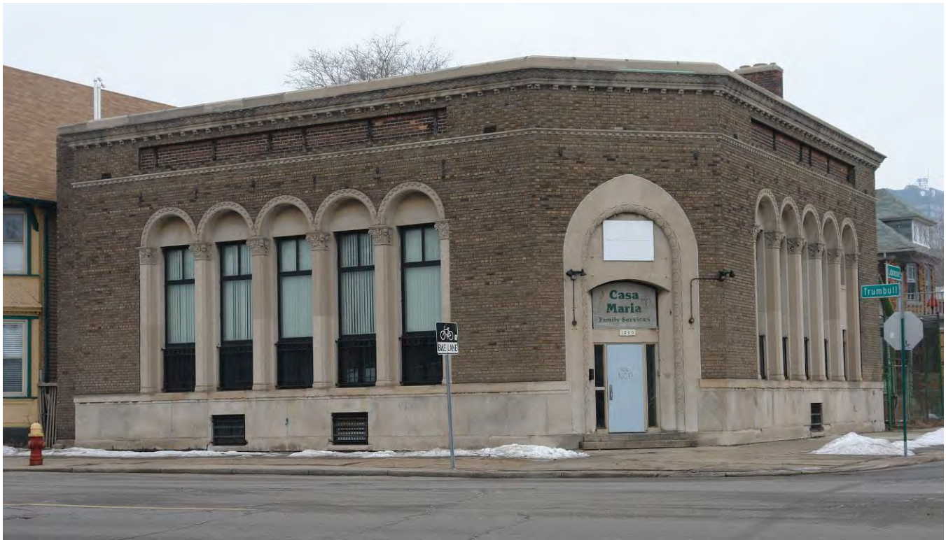
Figure 50: The Wayne County and Home Savings Bank branch at 1500 Trumbull Avenue and LaBrosse.
