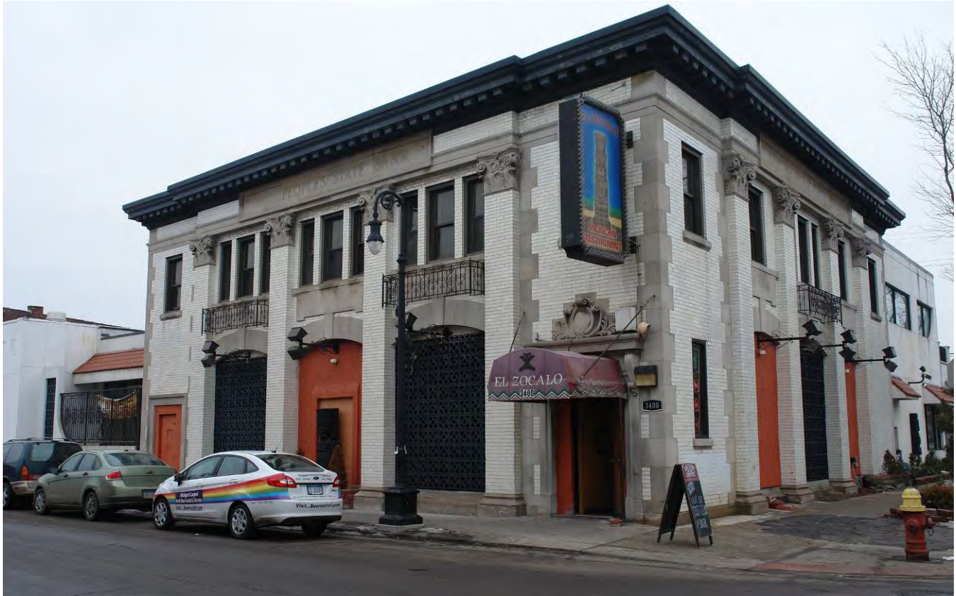
Figure 58: The Peoples State Bank branch at 3400 Bagley Avenue and 23 rd Street.
