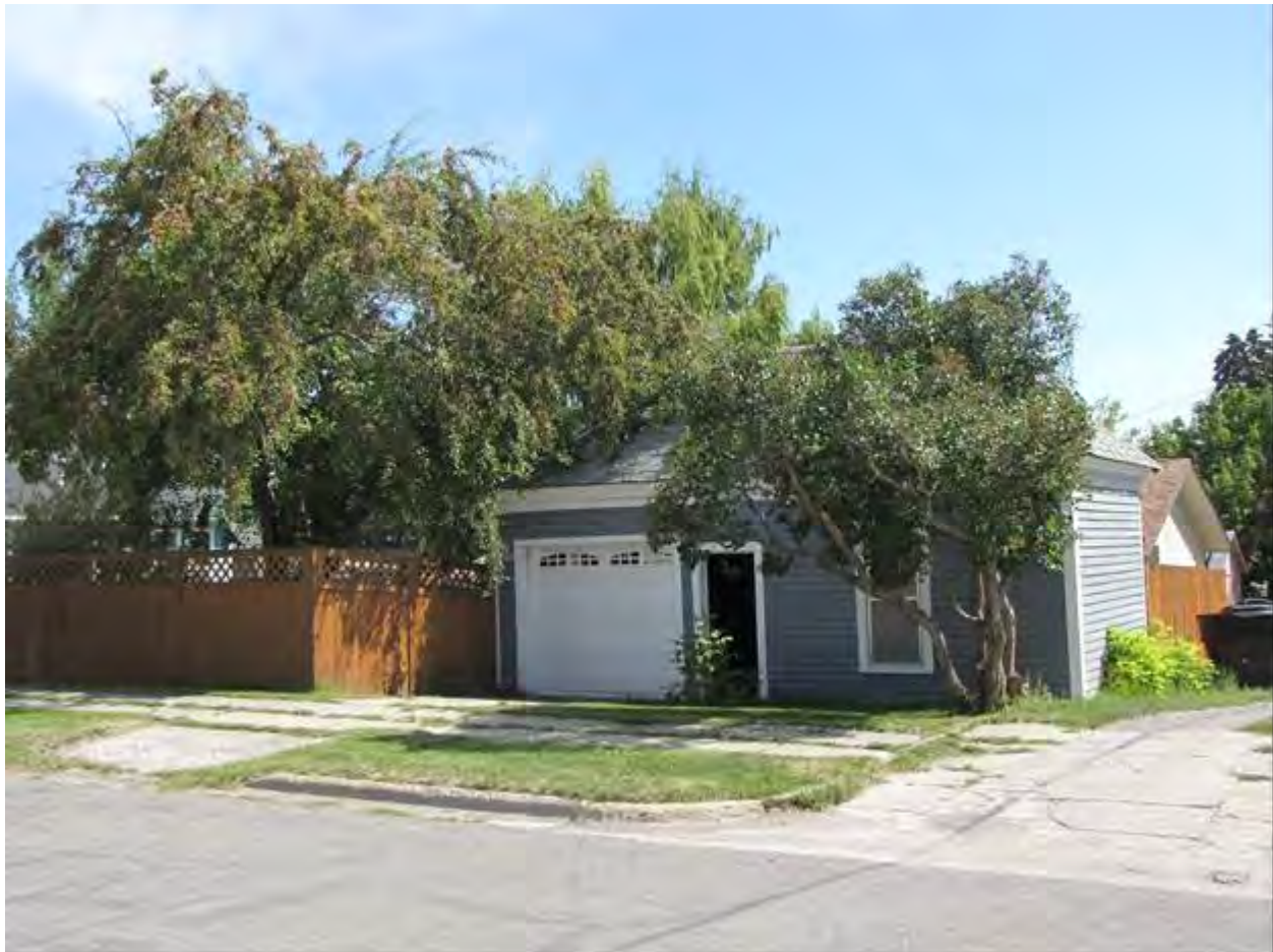
MT_LewisAndClarkCounty_Crump-HowardHouse_0009, Rear House, west and south walls, view to NE
