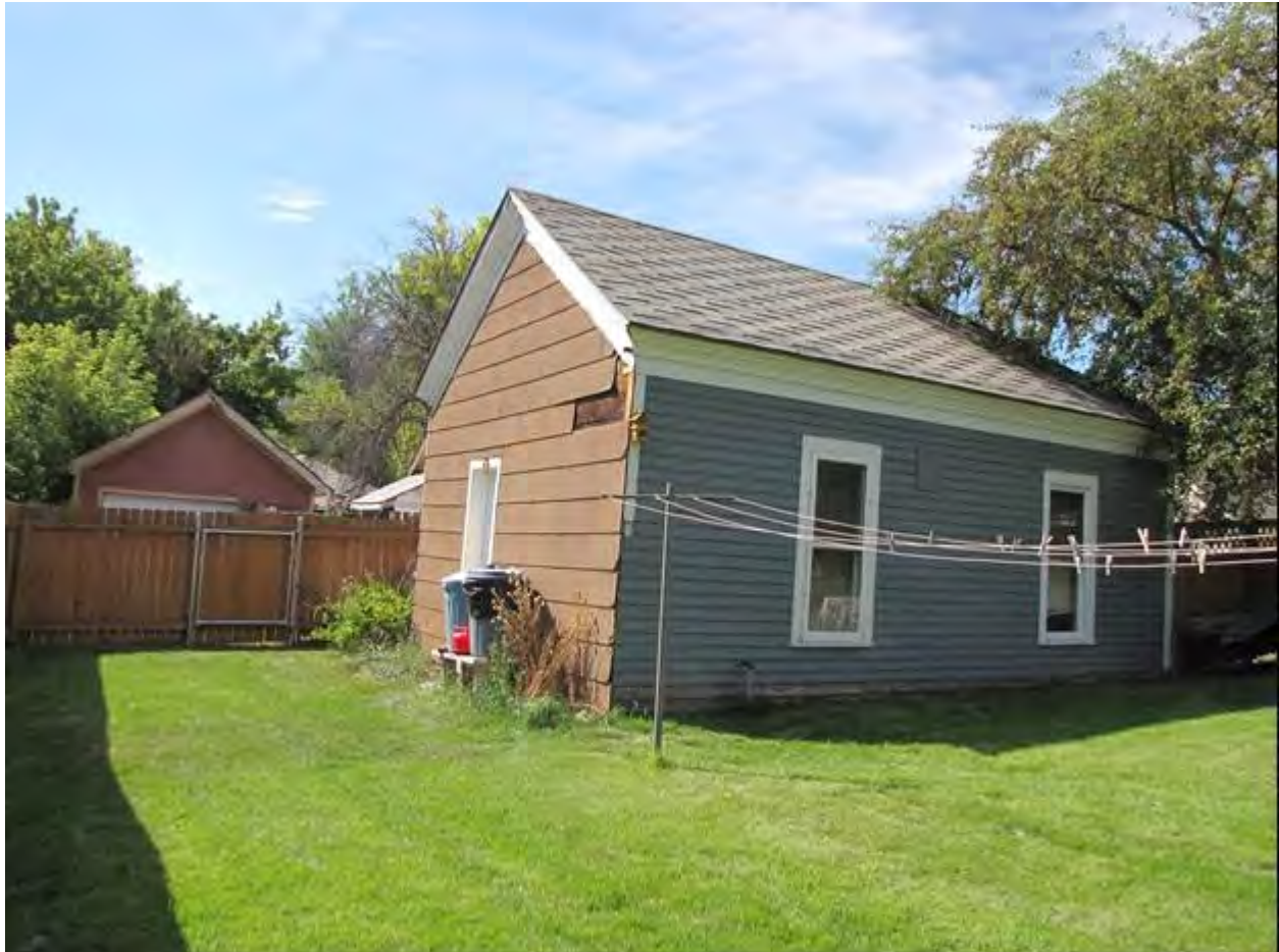
MT_LewisAndClarkCounty_Crump-HowardHouse_0011, Rear House, east and north walls, view to SW
