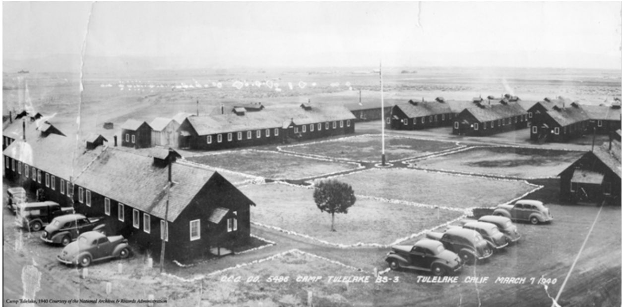
Figure 1. CCC Camp Tulelake, 1940. Extant barracks, top right; extant mess hall, center.
