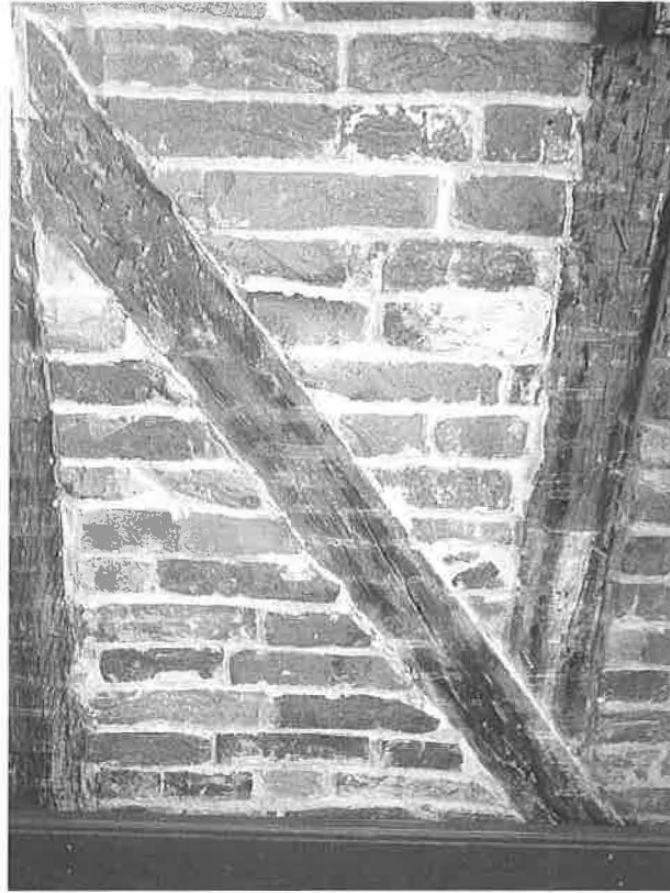
Image 7. Detail of half timbering with brick nogging at interior of Zoar Canal Inn (1832).
