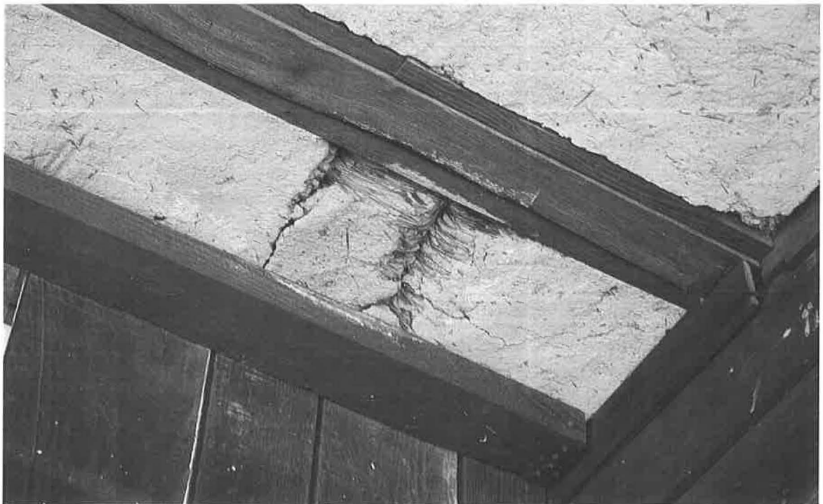
Image 8. View of Stroh-lehm paling insulation (Dutch biscuits) at rear façade of Zoar Store (1833).
