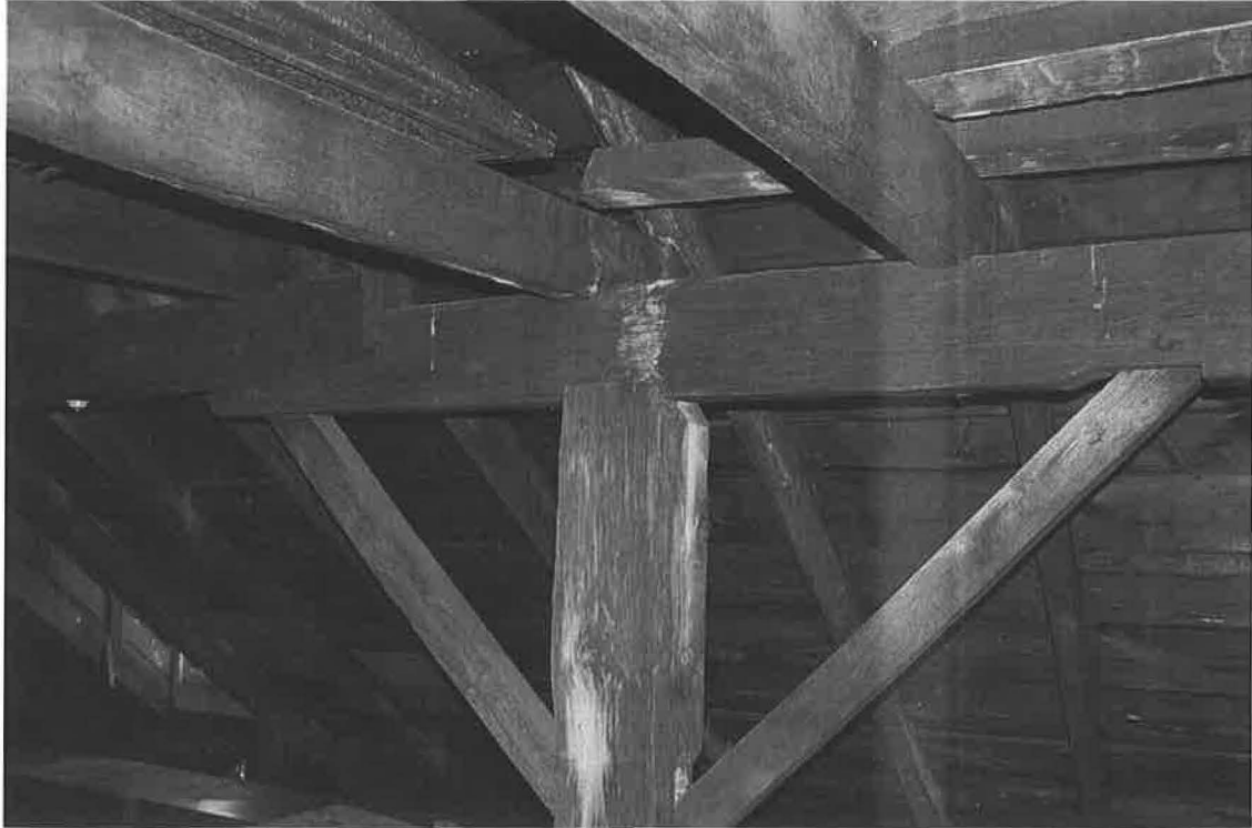
Image 5. Detail of post and beam construction in the attic of Number One House.
