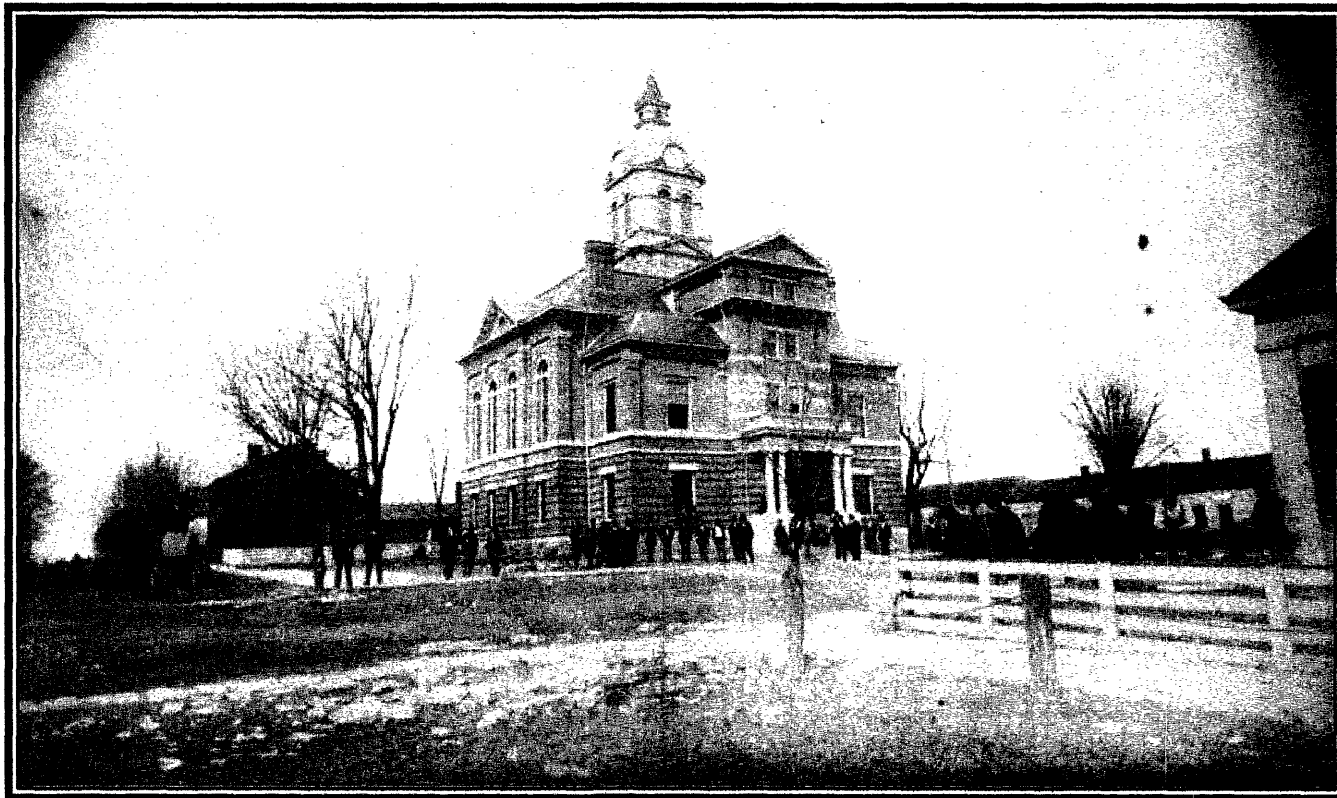
Fig. 4 The Court House as it was originally built had a large cupola which appears above in this c. 1890 photo. In the late 1890s, the roof began to sag from the weight of the cupola and Samuel Hannaford, Cincinnati's premier architect of the day, was called in to design a smaller cupola. The cupola depicted above was replaced
