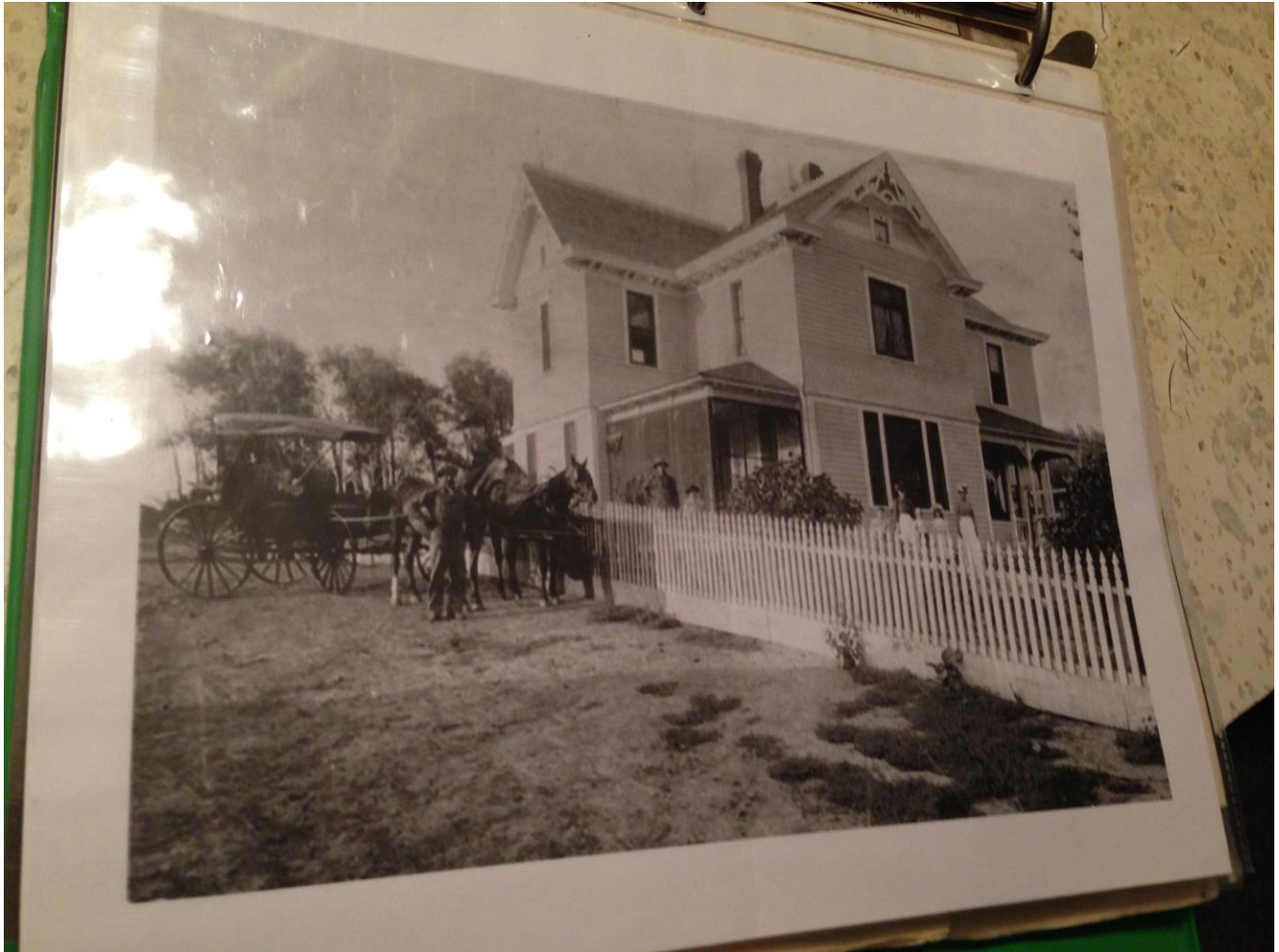
Figure 4: Historic photo of the farmhouse, date unknown. Many of the architectural details present in this photo, including the barge boards, bracketing, siding, and spindlework porches survive on the present house mostly unchanged.
