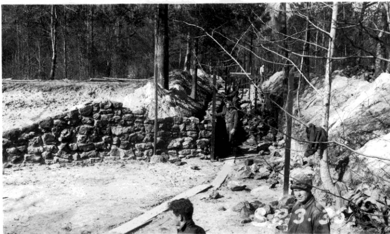
ROCK RETAINING WALL-----EAST END OF THE DAM NO. 35 SP-3 70
