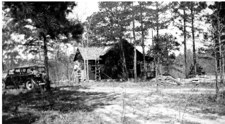
Figure 6: Cabin being stained [“Poinsett State Park (SP-3)--No.110 Overnight cabin, being stained, Project 107-B”, n.d. [ca. 1934-1942], Civilian Conservation Corps (CCC) files (photographs), State Commission of Forestry Records, South Carolina Department of Archives and History (SCDAH), Columbia, S.C.]
