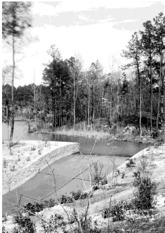
Figure 4: Large spillway showing concrete floor added by Company 2413. [Poinsett State Park Photograph Collection, SCDAH]
