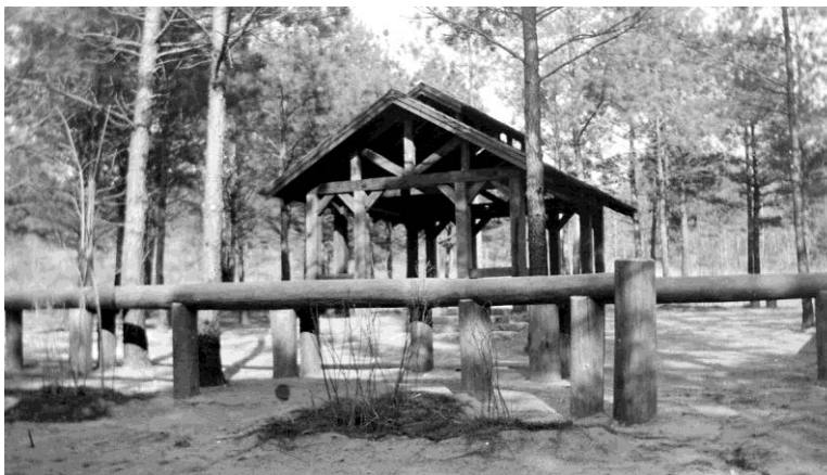
Figure 1: Picnic Shelter #2 [“Poinsett State Park (SP-3)—No.242 Guardrail at serving table, barbecue pit, and shelter: 5/1937,” May 1937, CCC files (photographs), State Commission of Forestry Records, SCDAH, Columbia, S.C.]
