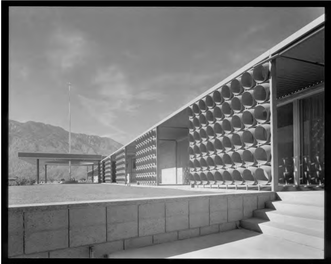
Figure 3. South elevation, looking west, 1958.
