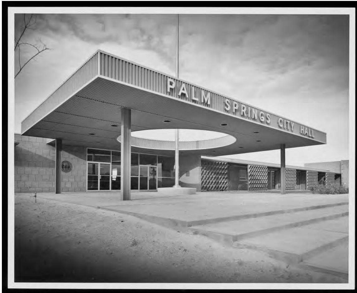
Figure 7. South elevation, looking northeast, 1958.
