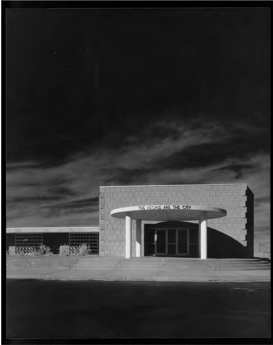
Figure 5. South elevation, council chambers, looking north, 1958.
