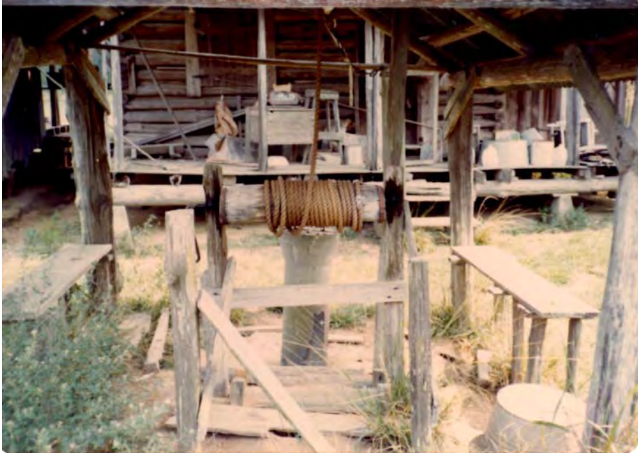
D. Historic well shed with curb well and winch in foreground and hand pump well behind.
