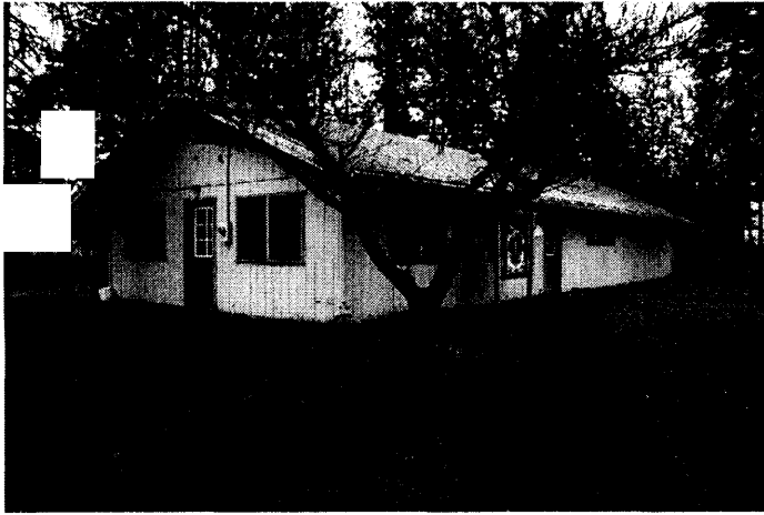
R-01: 1954 Barracks Photographer: Roger Brandt, 2005; Looking southeast Barracks constructed in 1954.
