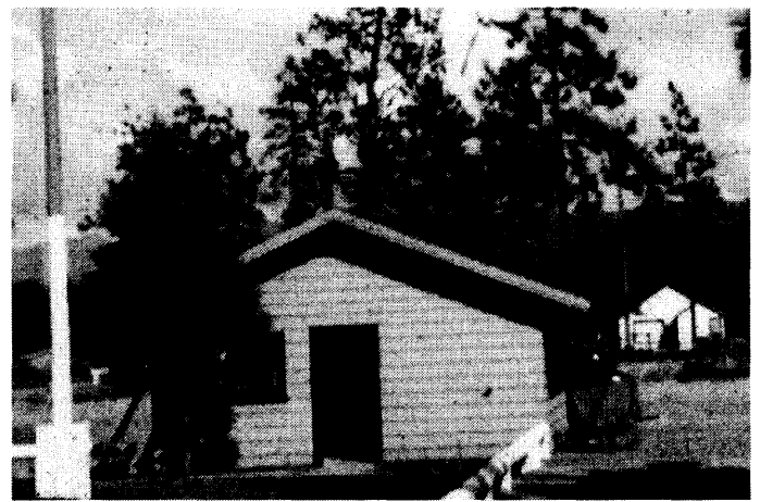
S-02: Storage shed Photographer: Jim Allen, circa 1952; Looking northeast Storage shed with the original shingle siding installed when the building was erected..
