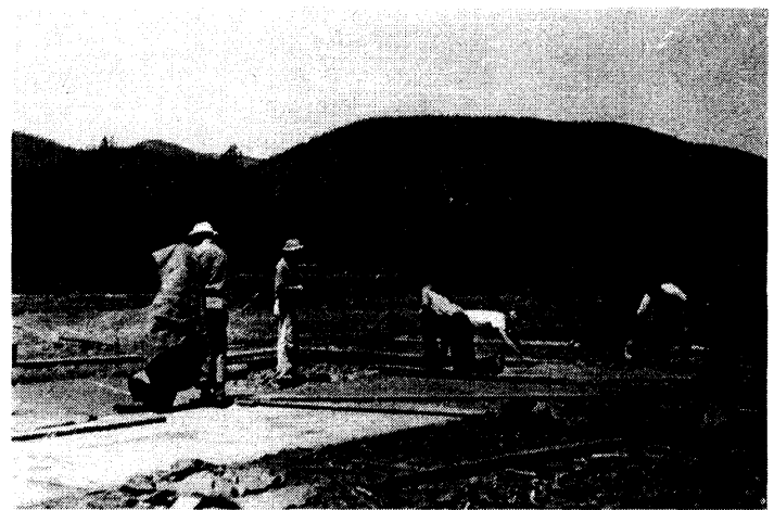
A-02: Construction of north warmup pad Photographer: Nick Pauls, 1945; Looking northwest. The pad was poured by the smokejumpers in the Civilian Public Service (CPS). Woodcock Mountain is in the distance.
