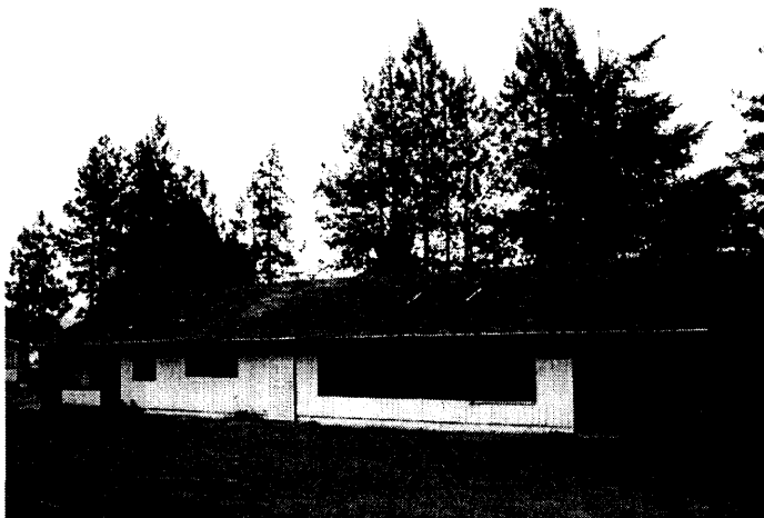
R-05: Cook house Photographer: Roger Brandt, 2005; Looking northeast This structure was reconstructed after fire damage in the early 60's. It sits on the same foundation and uses same entry walks.
