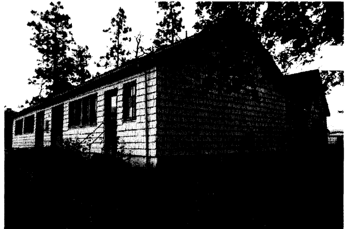
P-04: Parachute loft south and west walls Photographer: Roger Brandt, 2005; Looking northeast Dock and entrance to loft on left. Window of office has been removed and door added on west wall.
