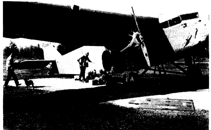
A-04: North warmup pad with metal fuel door Photographer: Bob Moffitt, 1948; Looking southwest. A metal fuel door is angled into the cement warmup pad. A smaller hinge door is seen along the left.
