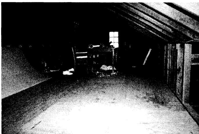
P-07: Parachute loft attic Photographer: Roger Brandt, 2005; Looking north A section of the attic above the repair room looking toward stair well. Storage bins can be seen along right.
