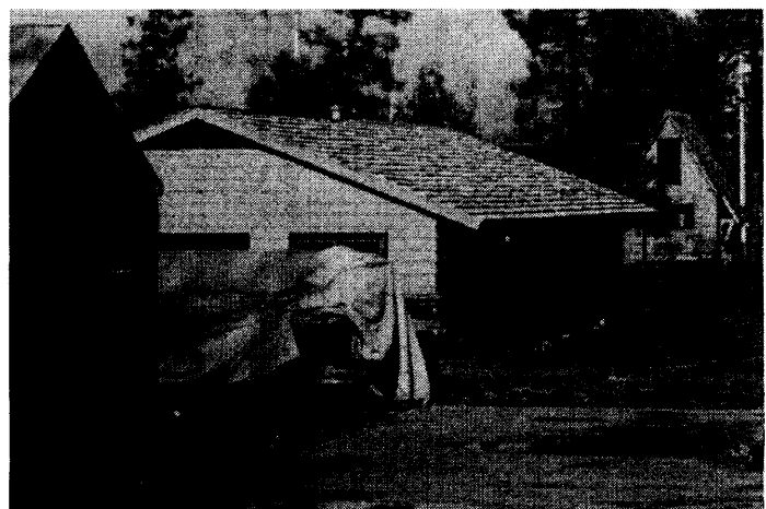
R-06: 1954 Cook house shingle siding Photographer: unknown, circa 1954. Looking north The original siding of the buildings constructed in 1954 were shingles. These were later replaced by plywood.
