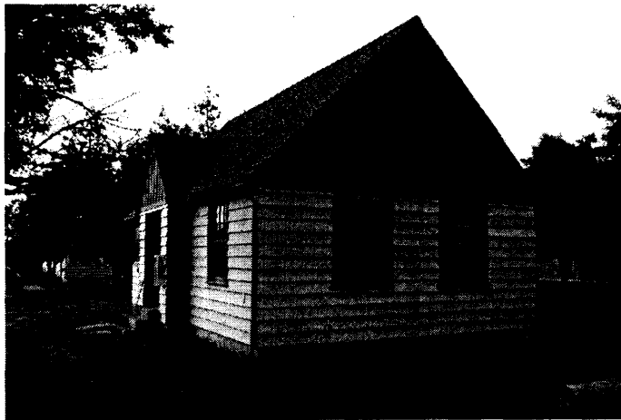
S-03: Administration office Photographer: Roger Brandt, 2005; Looking northeast The administration building was formerly the Redwood Ranger Station constructed in 1936.
