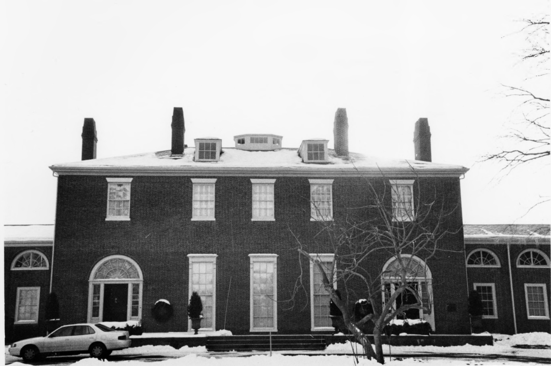
GORE PLACE Waltham, Massachusetts Front facade Photo: Robin F. Bachin, 1995
