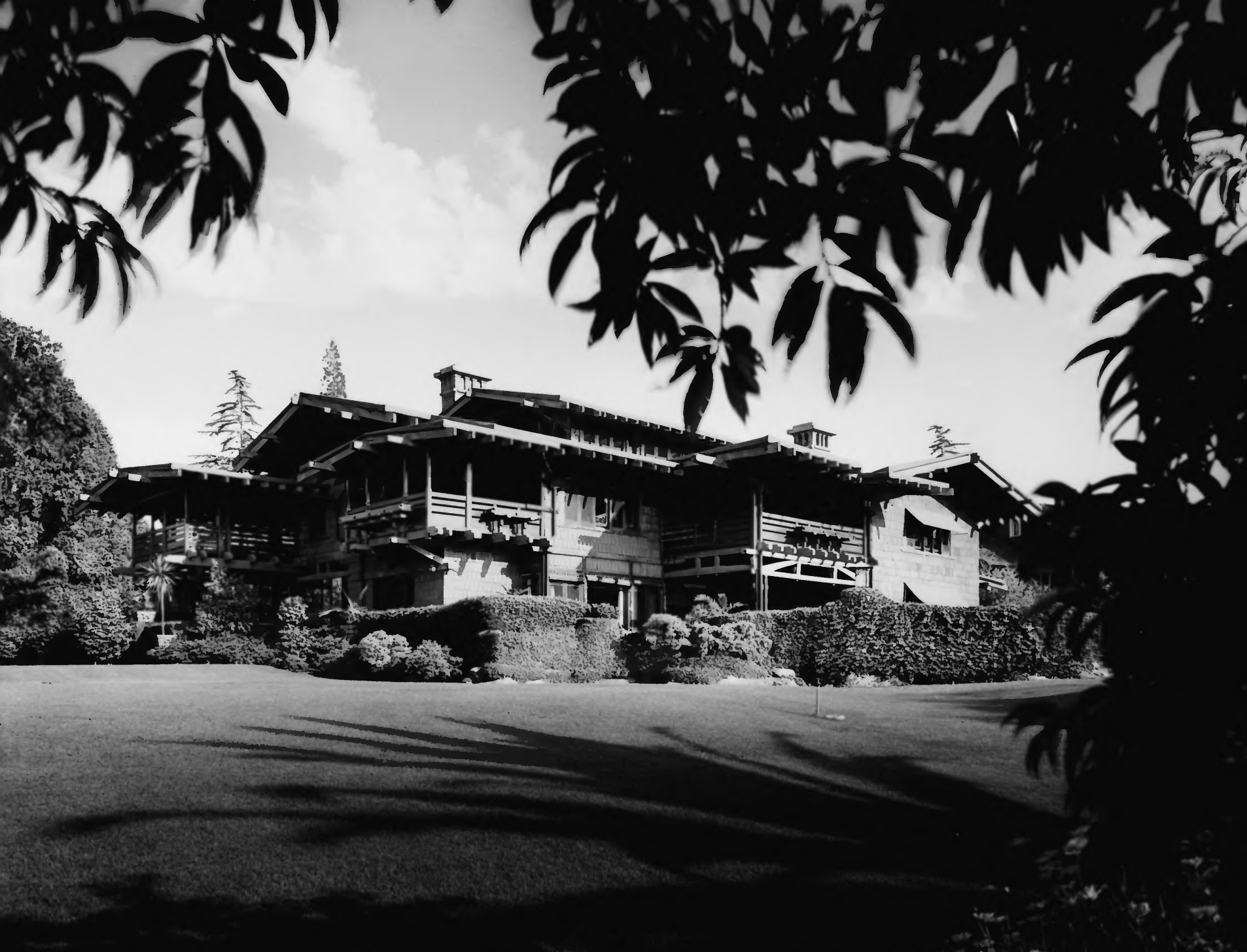
GAMBLE HOUSE, Pasadena, California; Photo Credit: Marvin Rand; Description: Rear View
