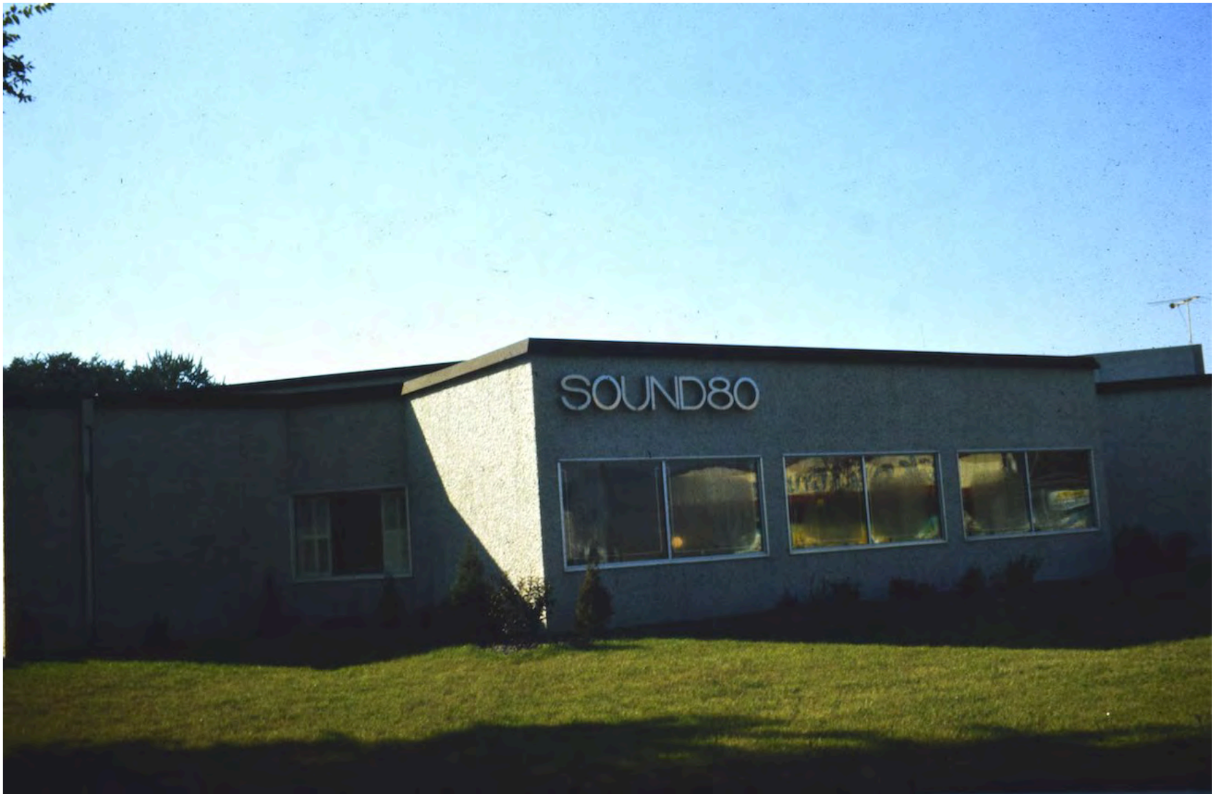
Figure 6. Sound 80 after completion of construction, circa 1971, facing south showing westernmost bay projection. Note coating, sign and windows.
