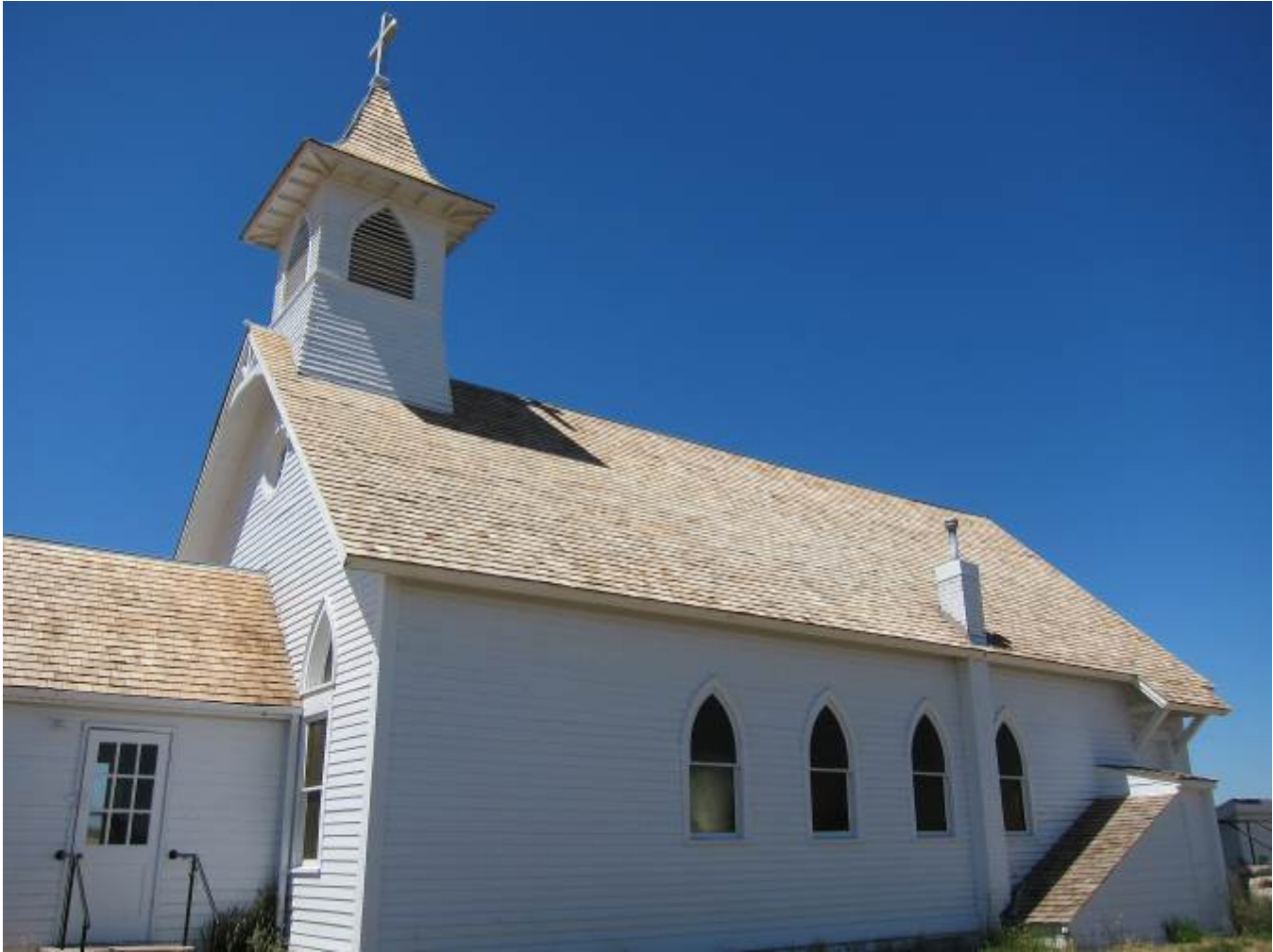
Photo# 0004: St. Wenceslaus Catholic Church, east elevation, view to northwest.
