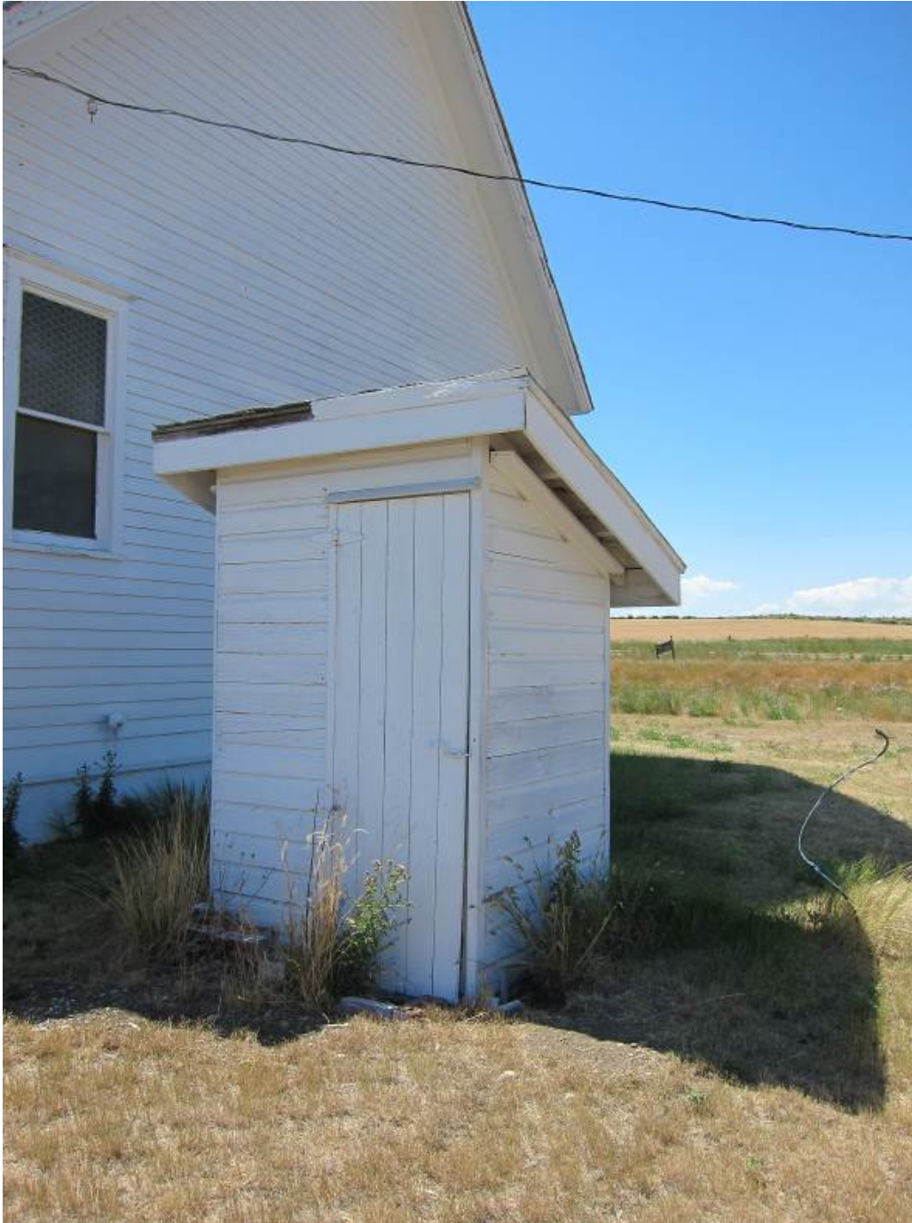
Photo# 0005: Outhouse, east and south elevations, view to west.
