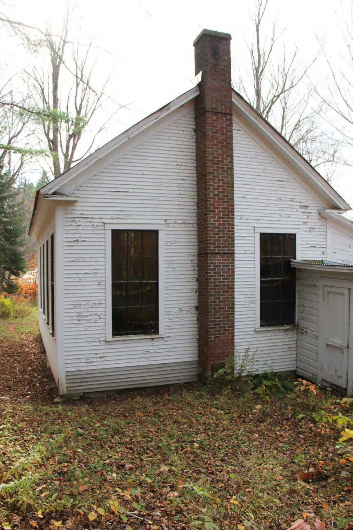
Beaver Meadow School, Norwich, Windsor Co., Vermont Photograph #10 of 16 Beaver Meadow School rear (north) elevation, view looking south
