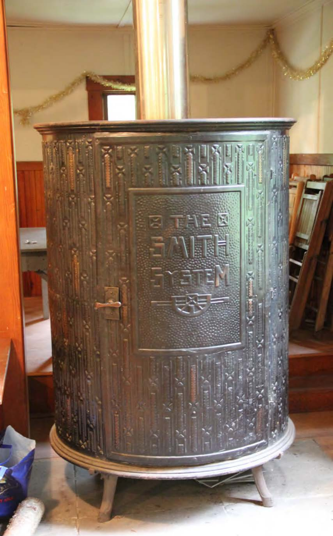
Beaver Meadow School, Norwich, Windsor Co., Vermont Photograph #16 of 16 Detail of jacketed "Smith System" stove
