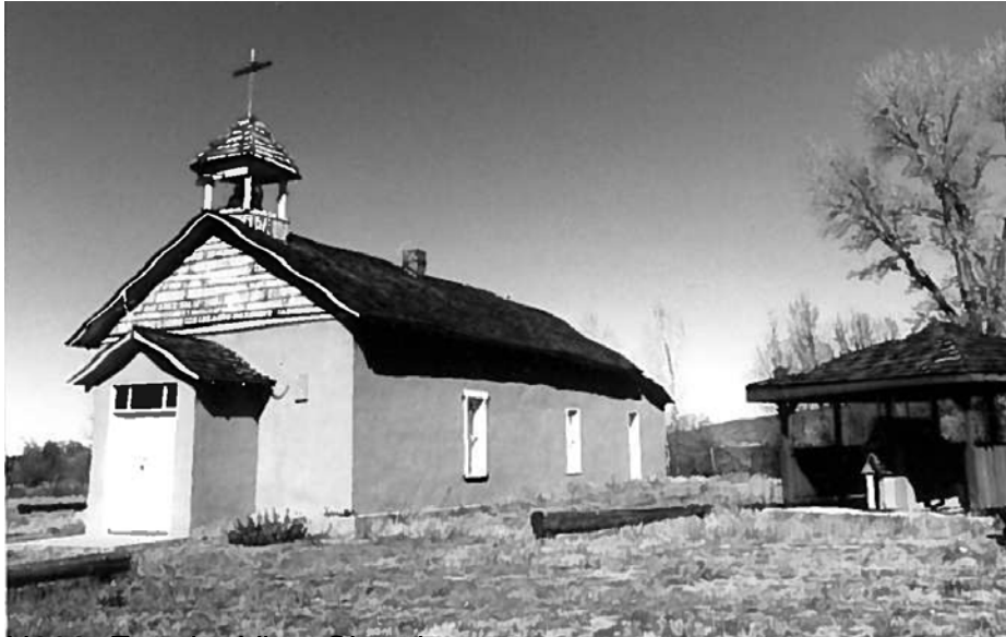
H003. Exterior View Church.
